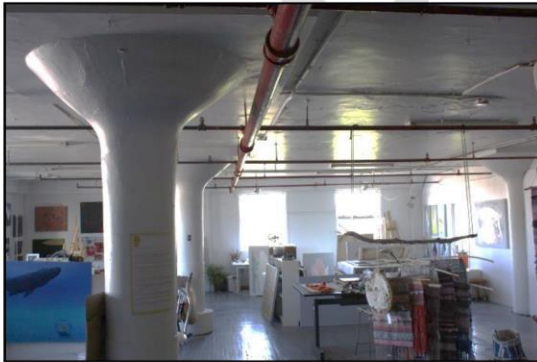
Photo 2: Typical columns inside the building [JCAL 2018].
