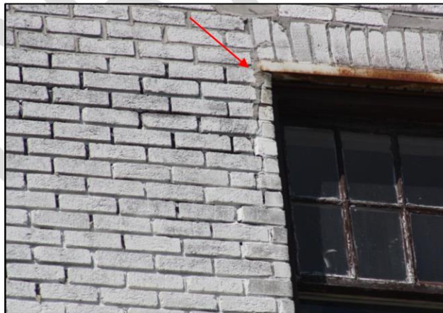
Photo 6: Third floor window on east elevation with deteriorated bricks around the perimeter [JCAL 2018].
