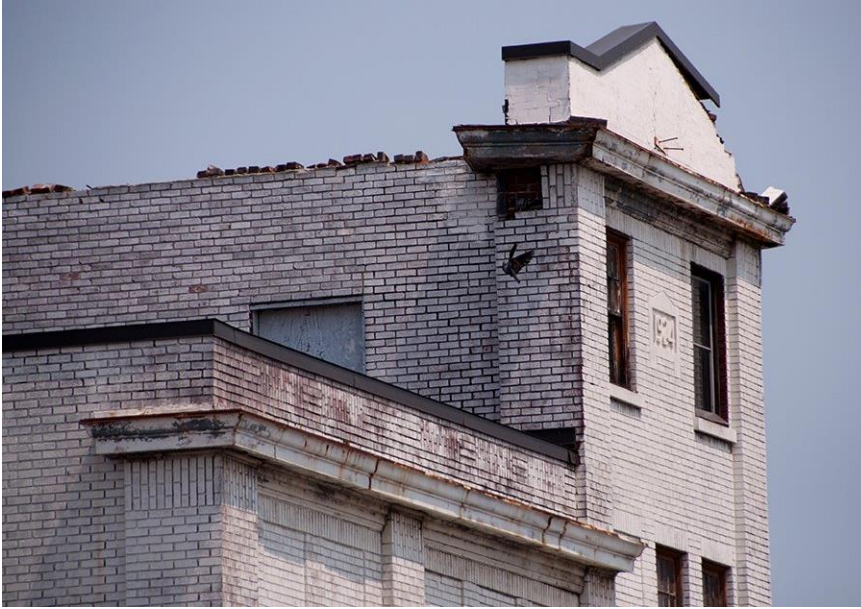
Figure 30: The gabled brick and metal parapets will be re-instated to their original form and design. The height of the parapet can be determined from period photos. The original colour of the brick is evident in areas where the paint has worn off. Bricked-in windows will be opened and reglazed retaining the glazing pattern.
