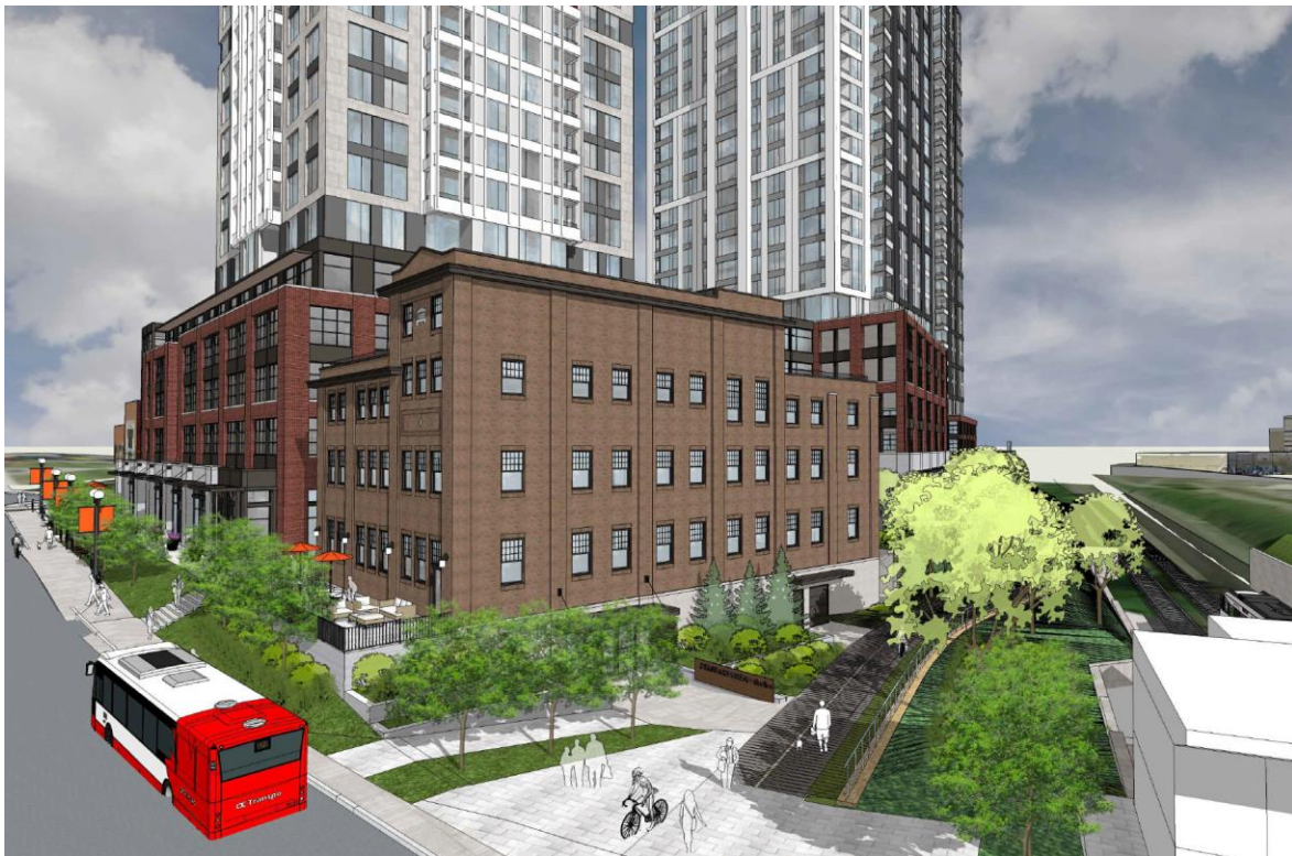
Figure 21: The view with public realm frontage on three sides of the complex set close to the street line on Gladstone. Ground floor retail has direct access. Source: Hobin Architecture 2022.
