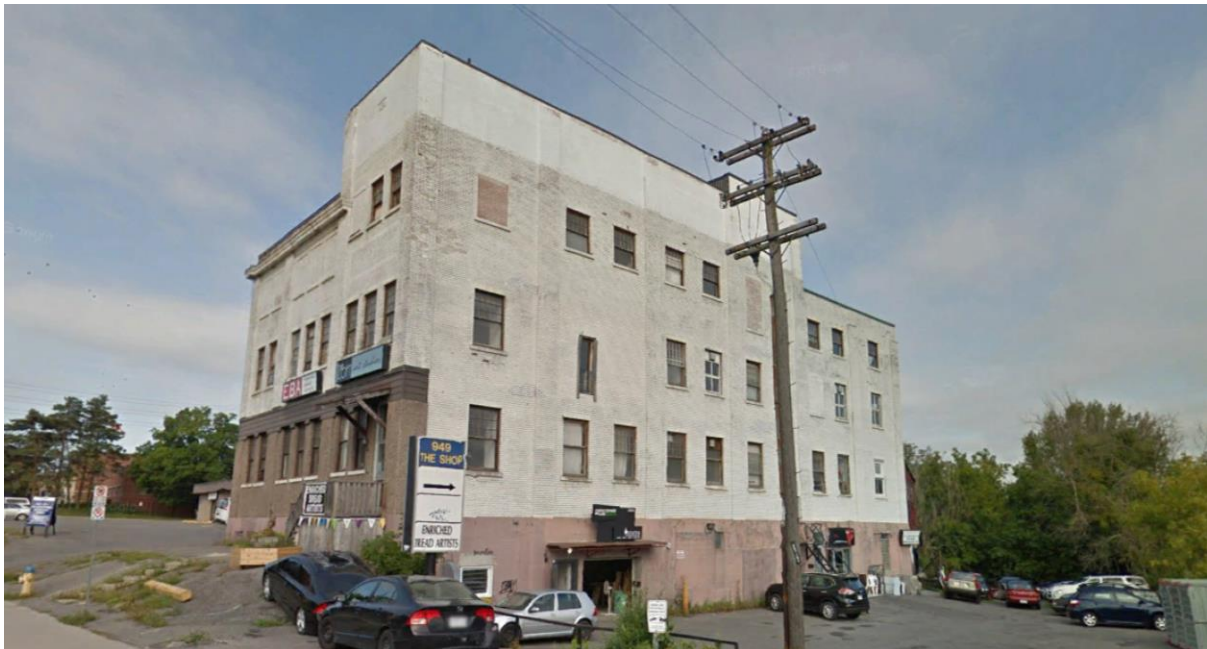
Figure 3: View looking west along Gladstone to the development site. Note the fenestration pattern on the east elevation (left) which characterizes its light industrial use with doors occurring on the second and third-floor levels and the location of an internal hoist to move material between floor levels. Source: Google Earth.
