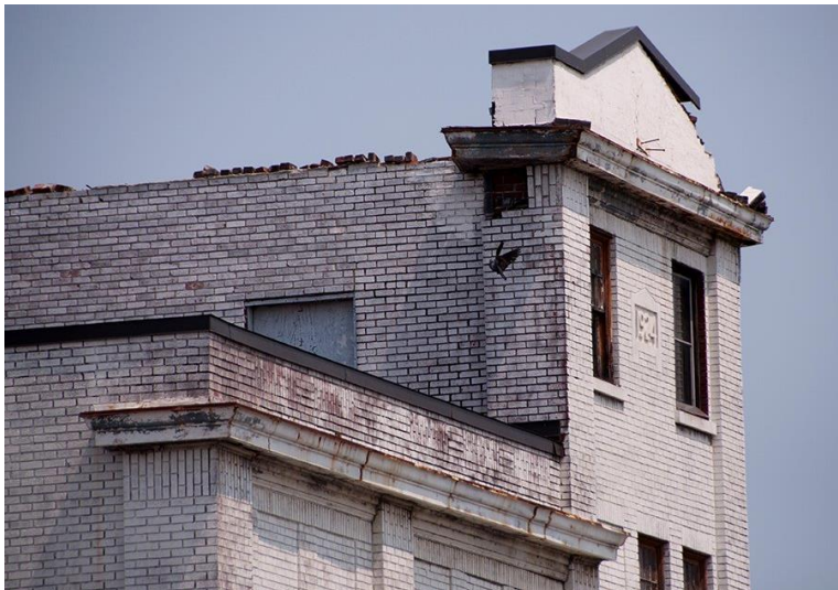
Figure 18: The gabled brick and metal parapets will be re-instated to their original form and design. The height of the parapet can be determined from period photos.
