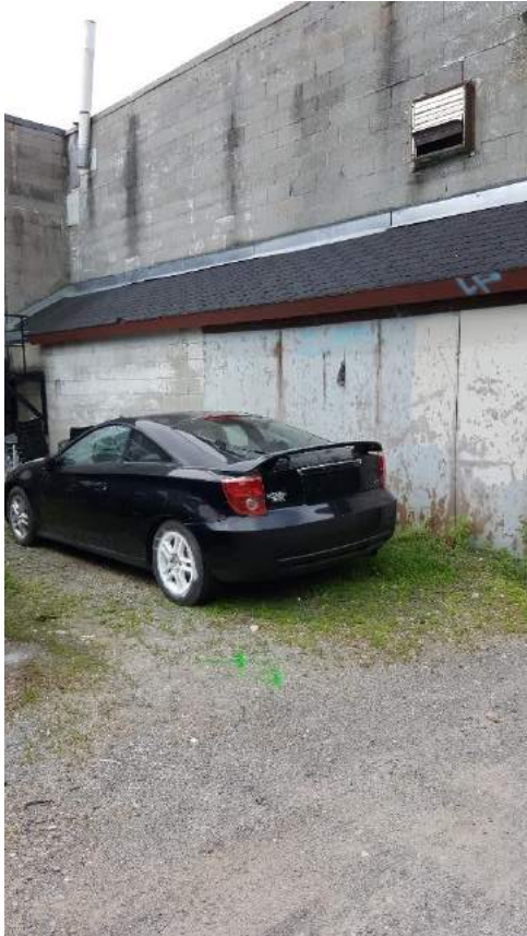
5.1 BH2017-5 Location moved three meters West
