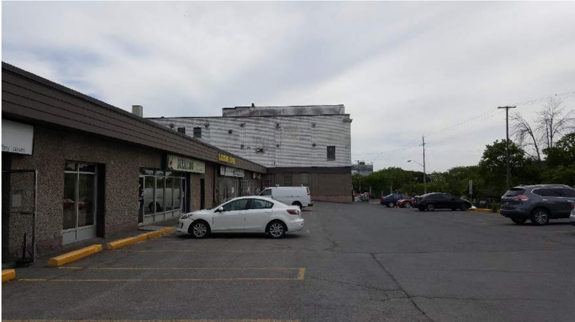
2.1 BH2017 – 2 Location, looking East.
