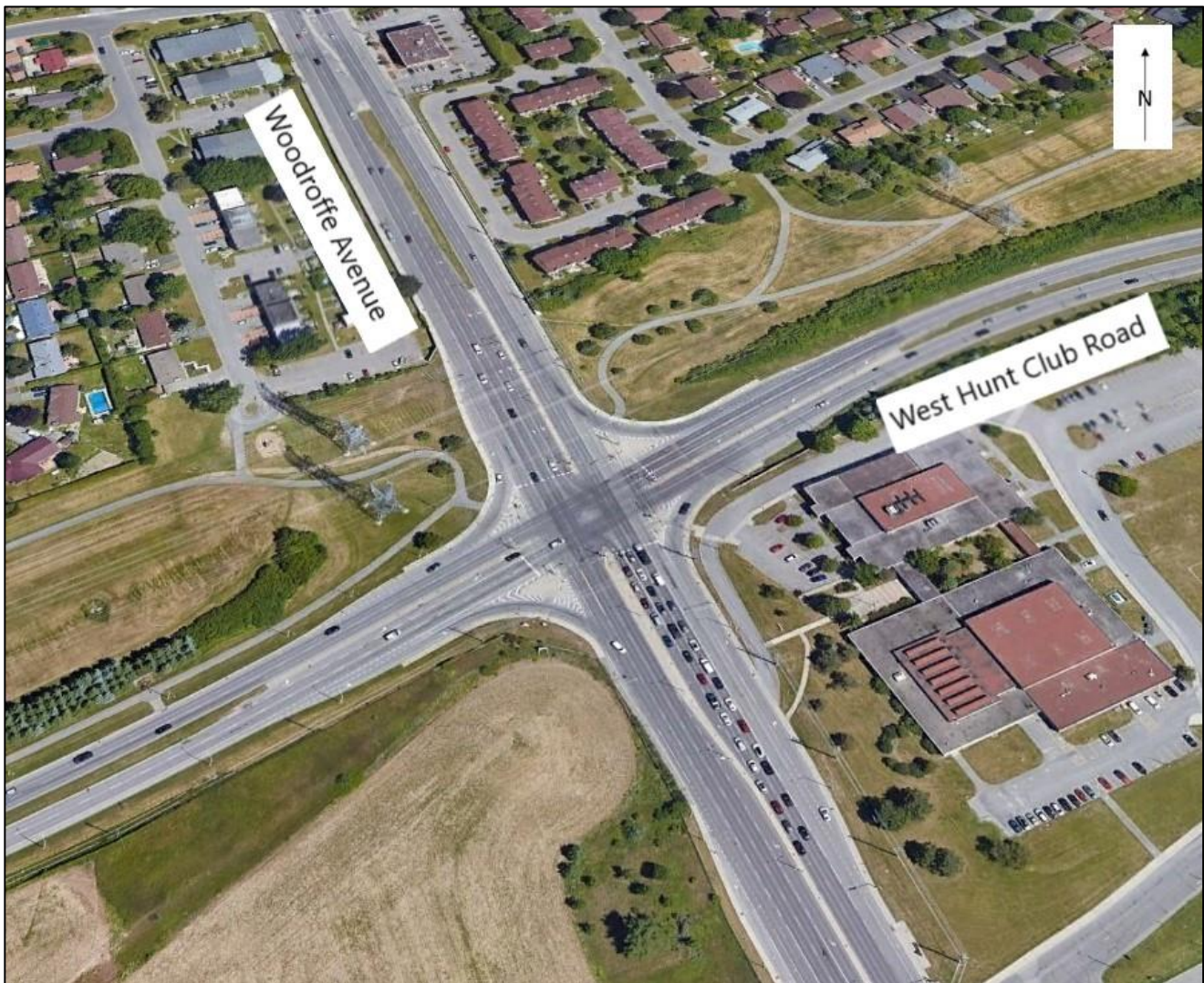
Figure 3.1 Woodroffe Avenue at West Hunt Club Road
