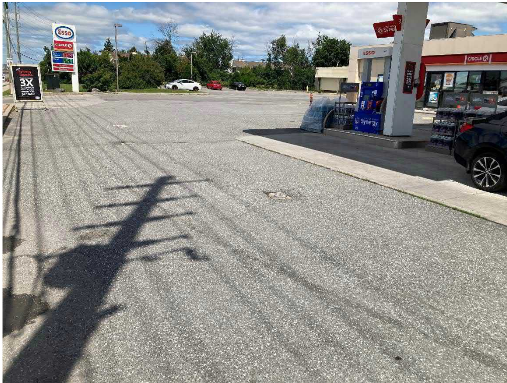
Photo 9: View of monitoring wells installed west of the fuel pumps
