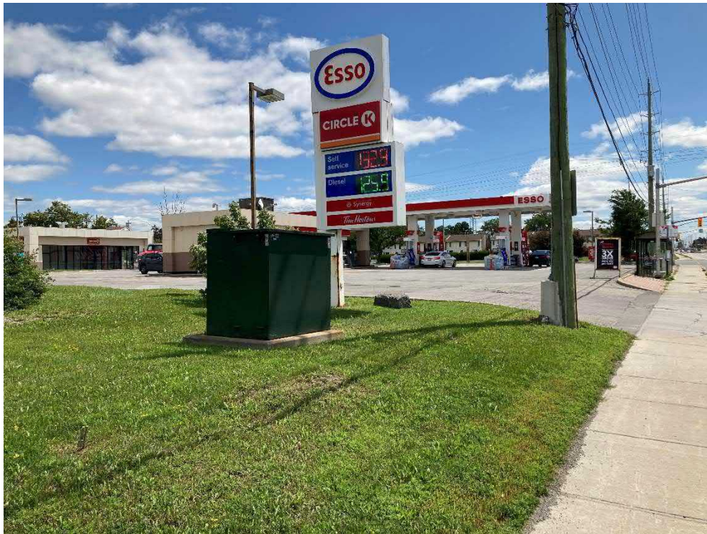
Photo 3: View of the retail fuel outlet, car wash (background) and transformer box (foreground)
