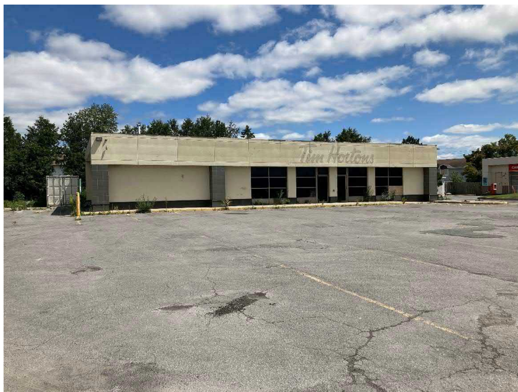
Photo 6: View of the commercial building in the northeast portion of the Site
