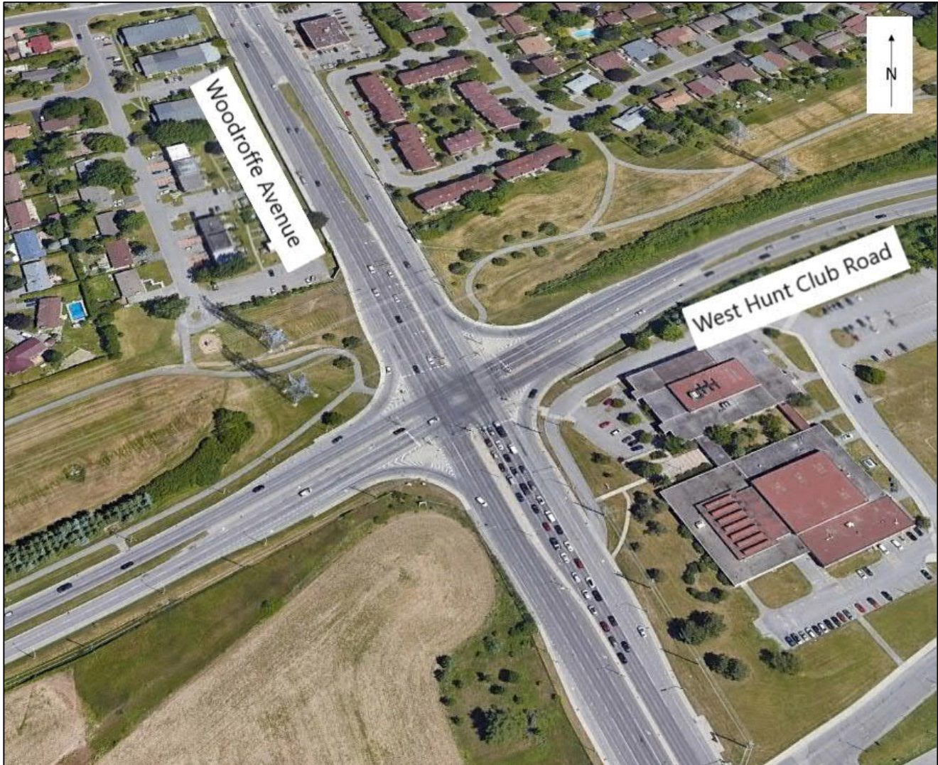
Figure 3.1 Woodroffe Avenue at West Hunt Club Road
