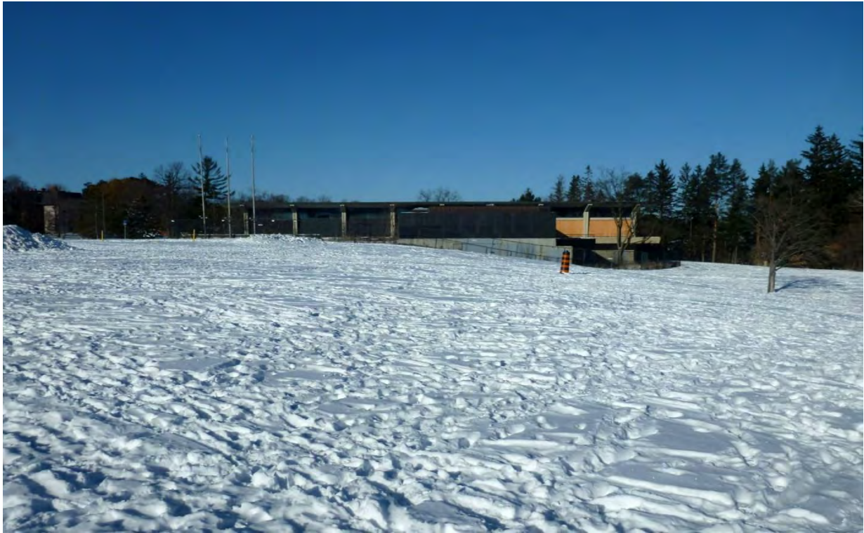
Figure 15: View of the Annex facing north
