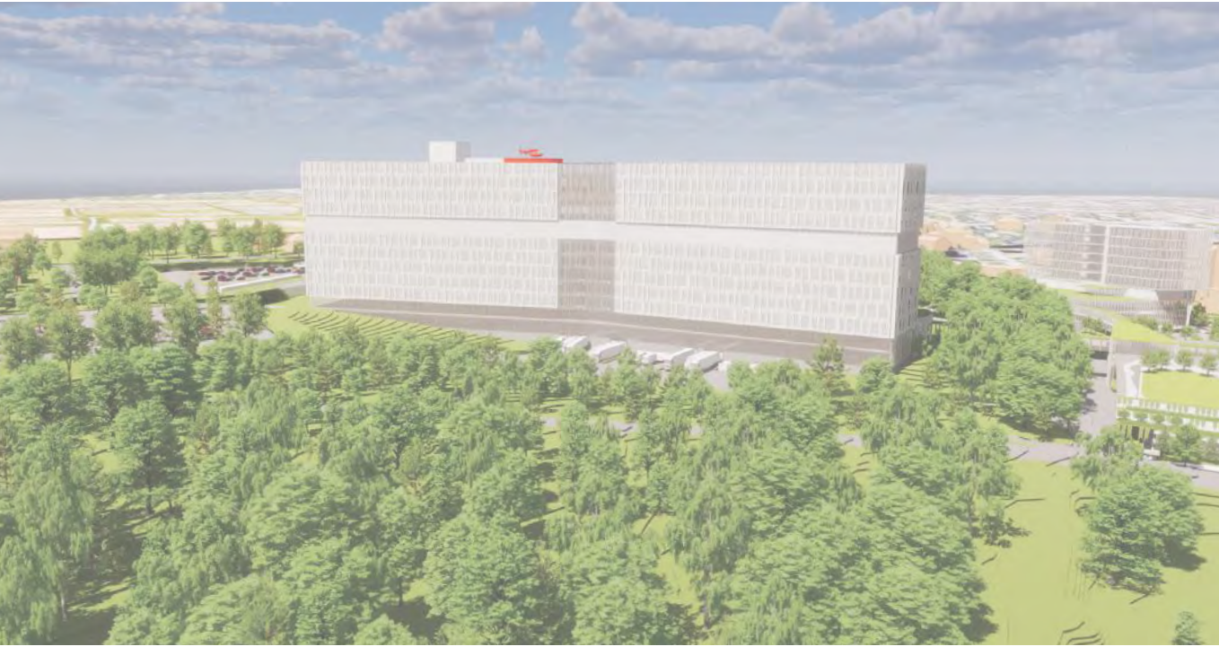
2 - PRINCE OF WALES DRIVE (facing west/south towards loading docks)
