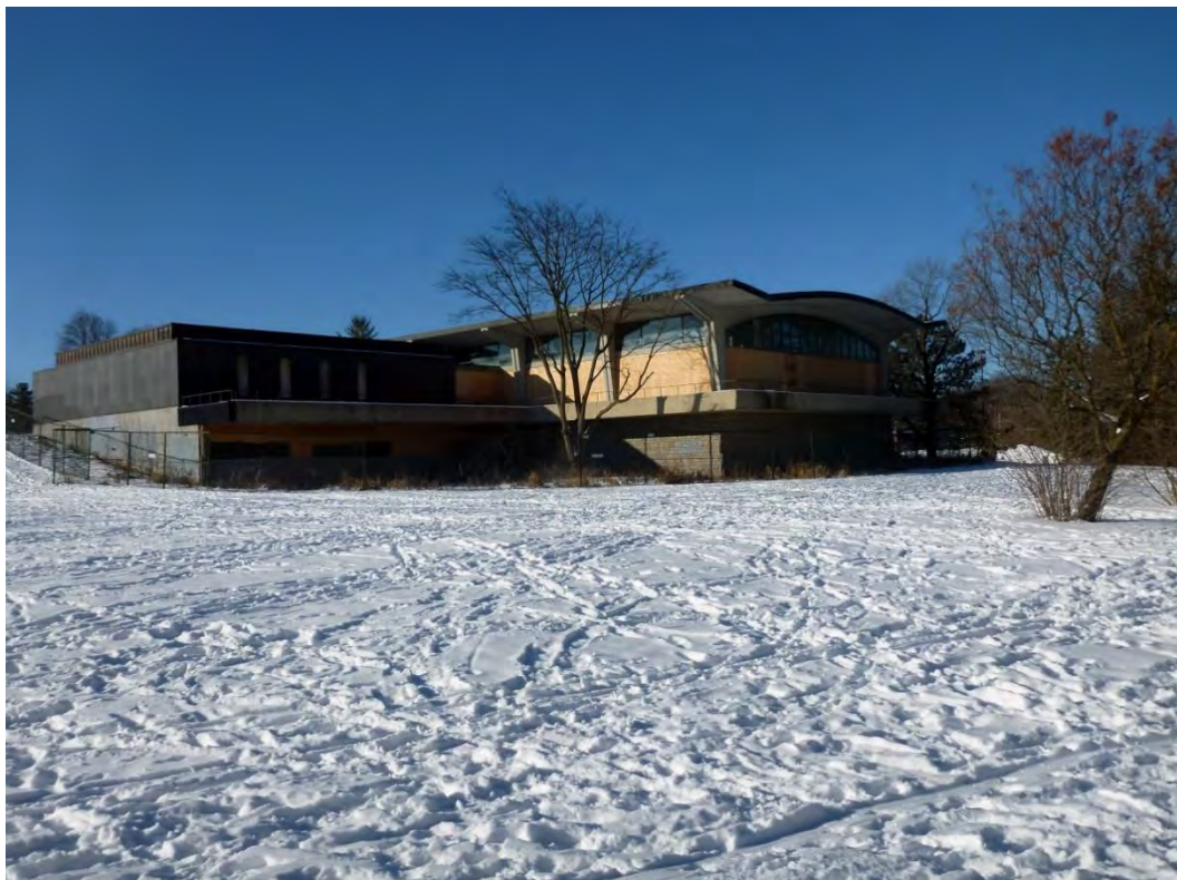
Figure 14: View facing west of the Annex
