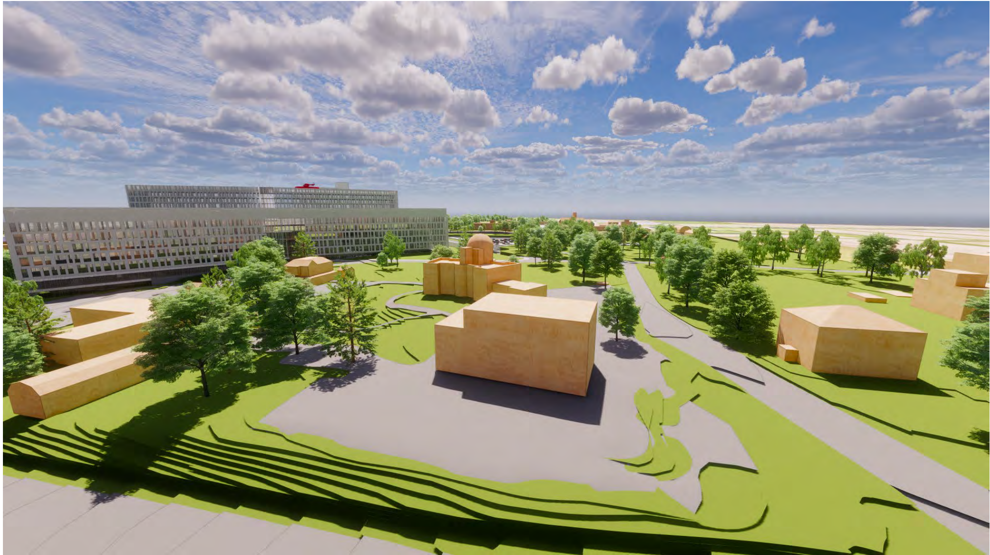
THE OTTAWA HOSPITAL – CIVIC REDEVELOPMENT PROJECT VIEW SOUTH FROM THE DOMINION OBSERVATORY CAMPUS (FOREGROUND)
