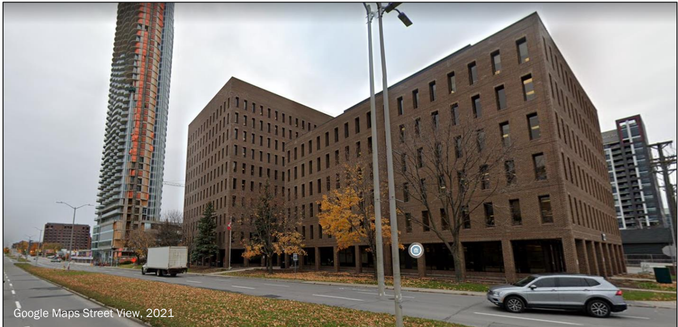
Photo 5: Mid-Rise Institutional and High-Rise Residential west of Rochester Street (looking northwest)
