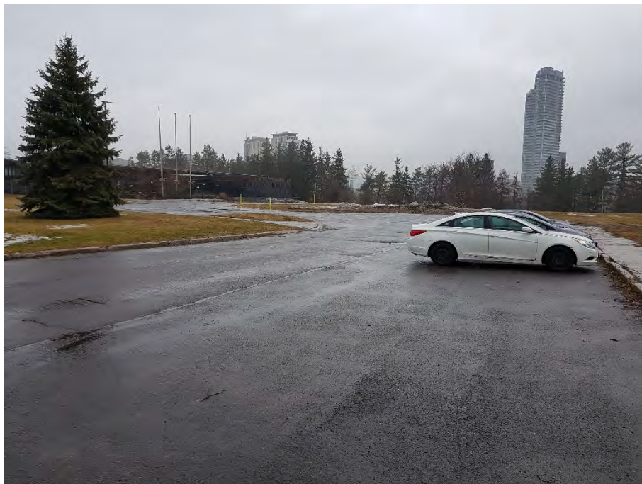
Image 6: Surviving parking lot south of the recently demolished Sir John Carling Building, view north. The cafeteria wing, all that remains of the building, is visible in the background.
