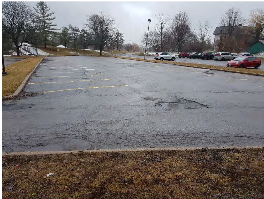
Image 4: Parking lot built for the recently demolished Sir John Carling Building, view southeast.
