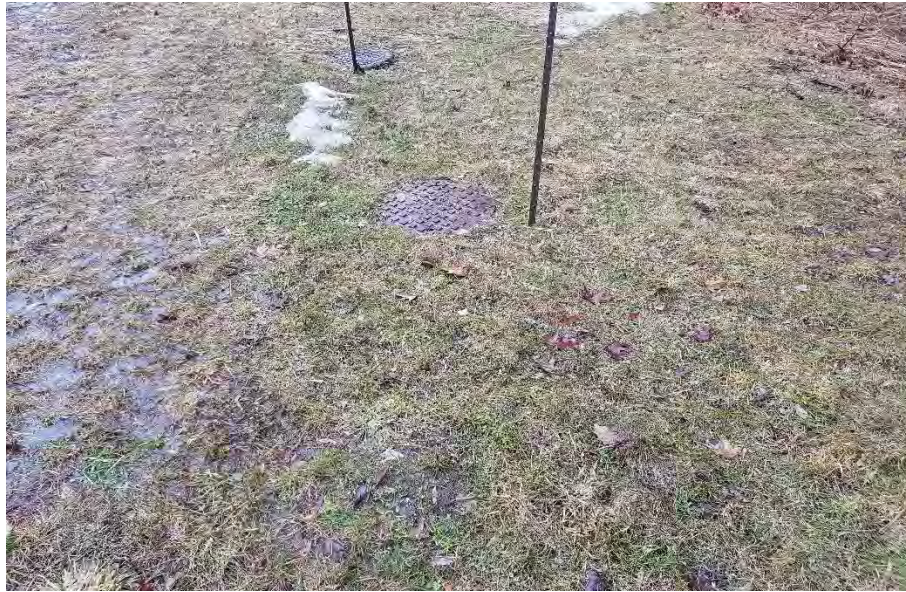
Image 5: Two man holes located north of the location of the former Sir John Carling Building showing the location of underground infrastructure, view northwest.
