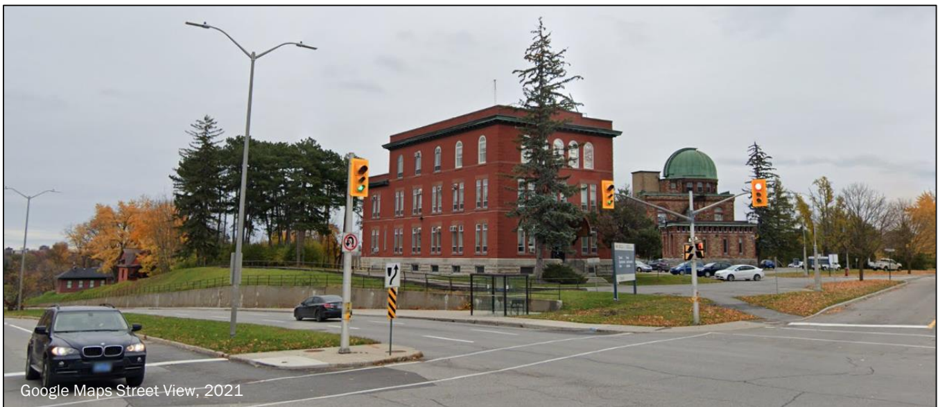
Photo 2: Low-rise buildings at Maple Drive (looking southeast)
