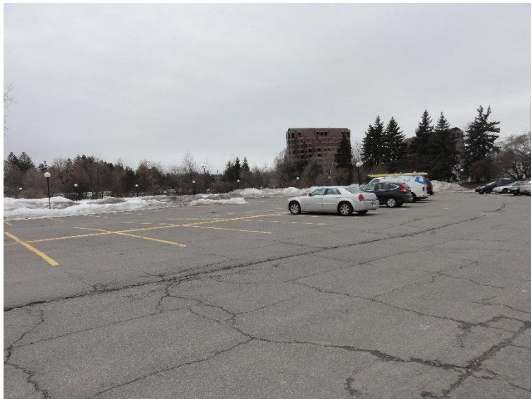
Photo 2 – View of northern portion of Parcel A occupied by a commercial parking area, looking northwest.
