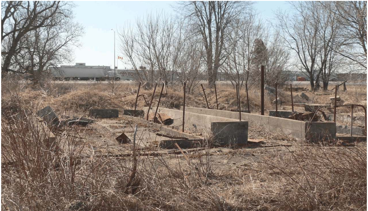
Plate 7: Remains of a concrete barn foundation (dairy cow stalls) near the southeast corner of the property (adjacent to BhFx-40). Note the piles of disturbed ground to the rear (east) of the building remains.
