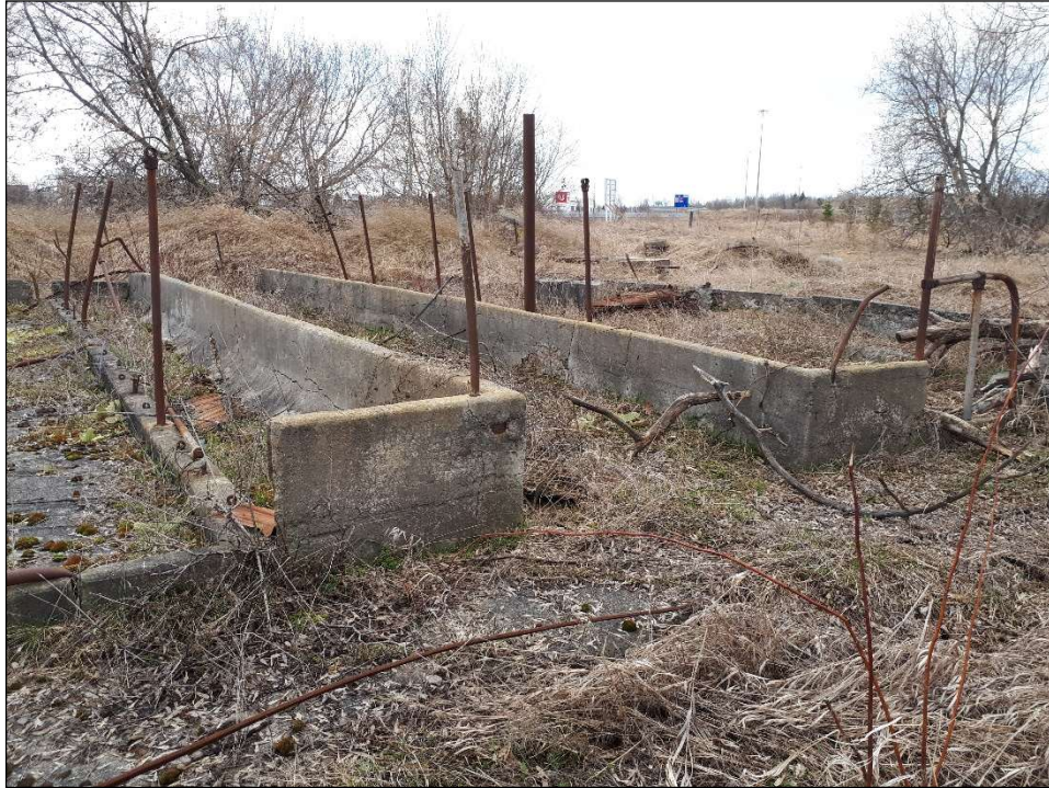
Photo 4: Former building foundation on-site.
