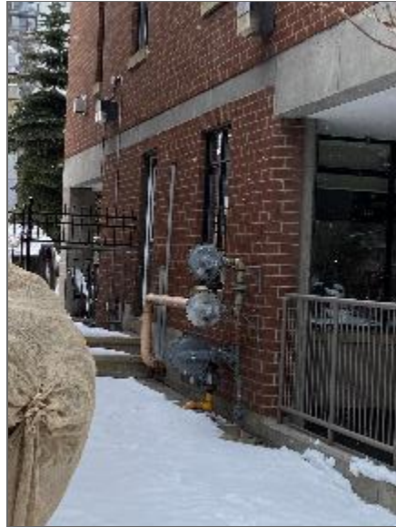
Photo 11 – Fill and vent pipes observed at 364 Cooper Street.
