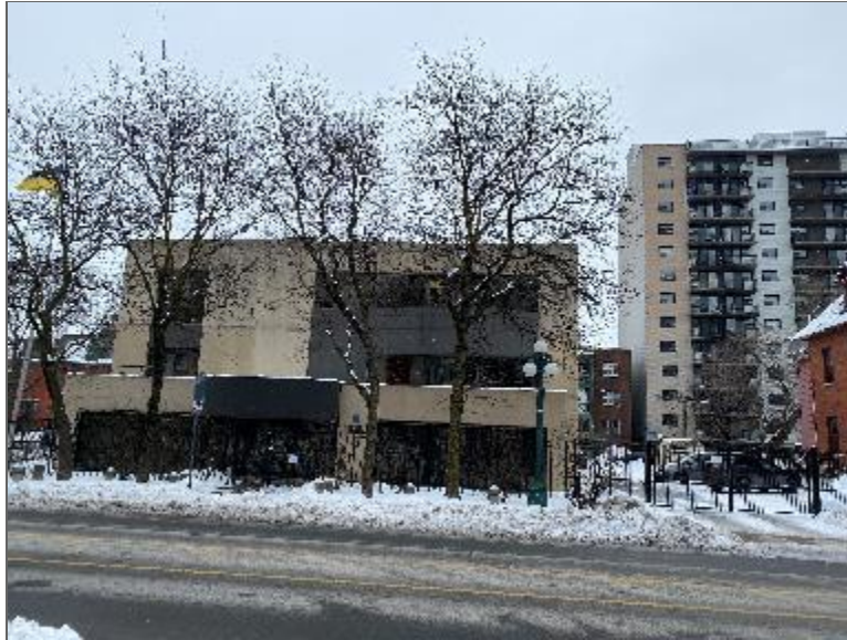
Photo 5 – Looking south from the Phase One Property across Somerset Street West.
