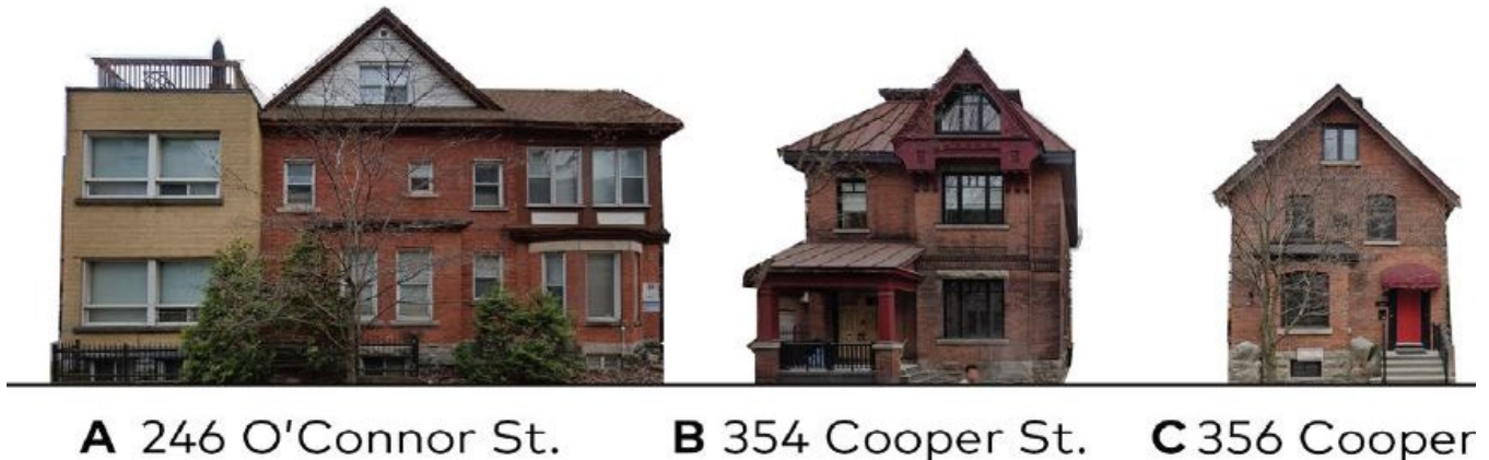
Figure 11 Heritage Considerations on Cooper Street.
