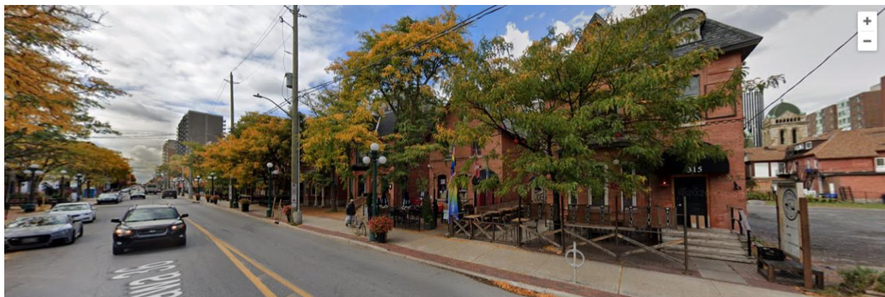
Figure 4: Context view of the site (left) with the adjacent buildings along Somerset St. Credit: Google Earth.
