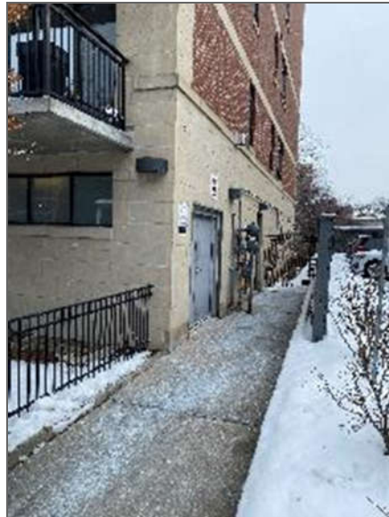
Photo 10 – Fill and vent pipes observed at 374 Cooper Street.
