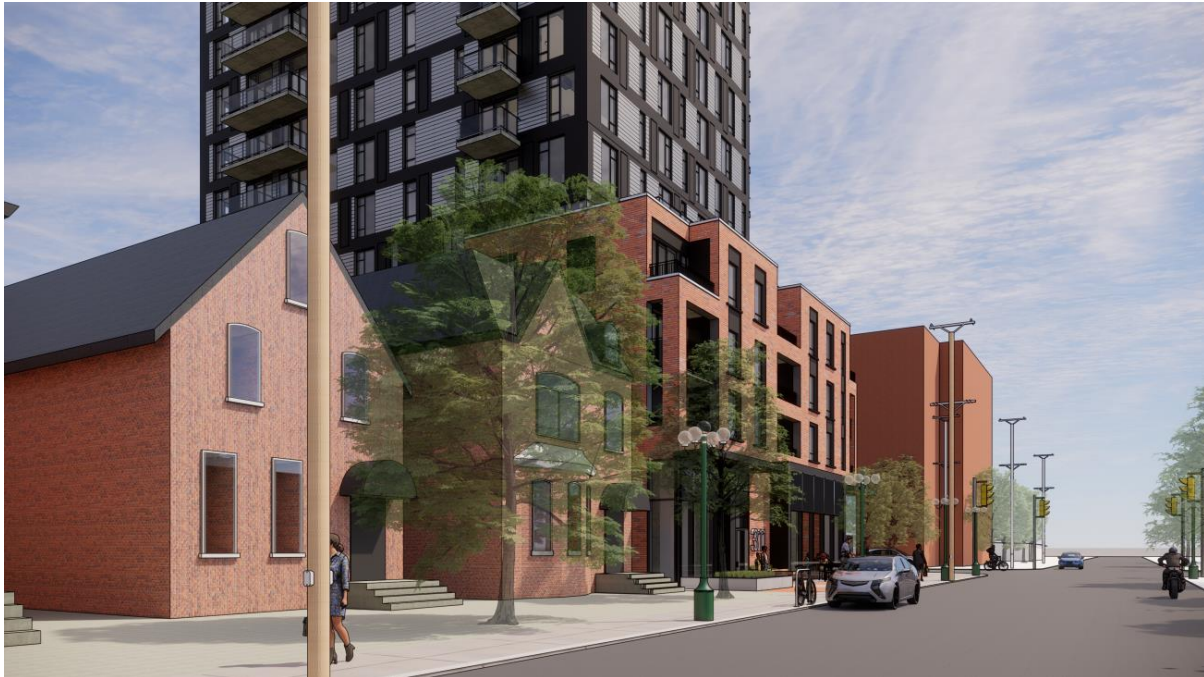
Figure 19: View looking northeast of the proposed development illustrates the stepping of the tower and the open balcony on the 4 th floor referring the height of the older homes along Somerset with the defined step backs and material changes of the tower. Source: Figurr Architects Collective.
