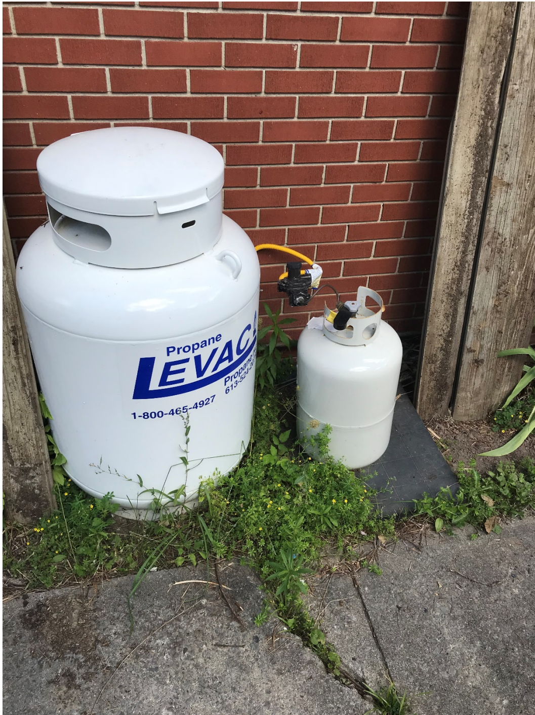
West exterior wall
