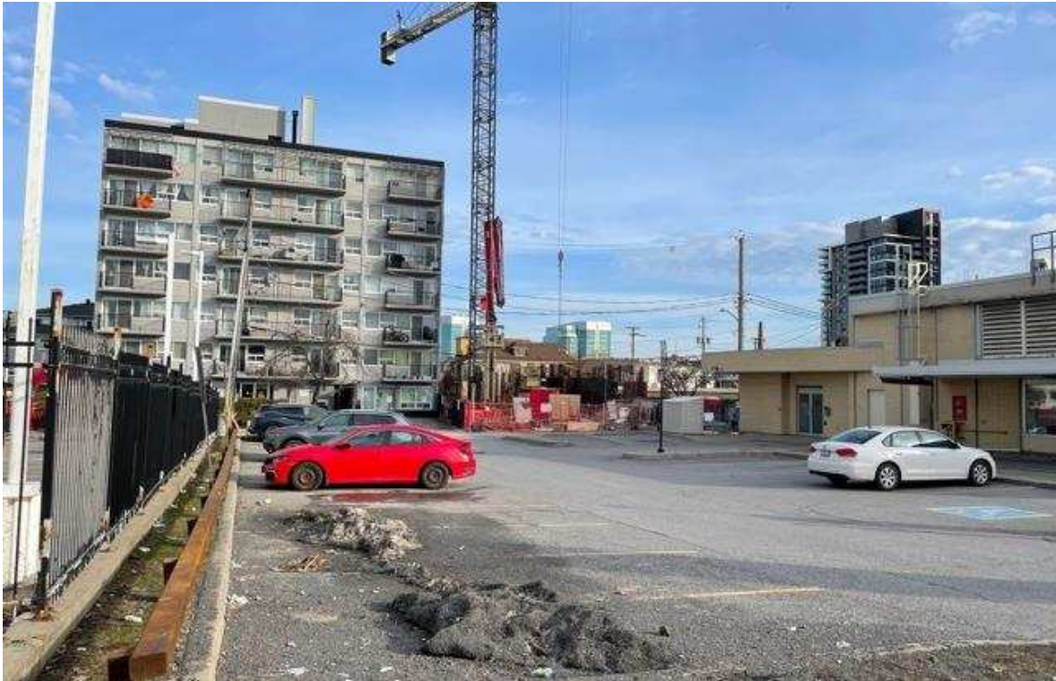
Photograph 2: View of the western half of the Phase I Property. Photograph taken from Carling Avenue.
