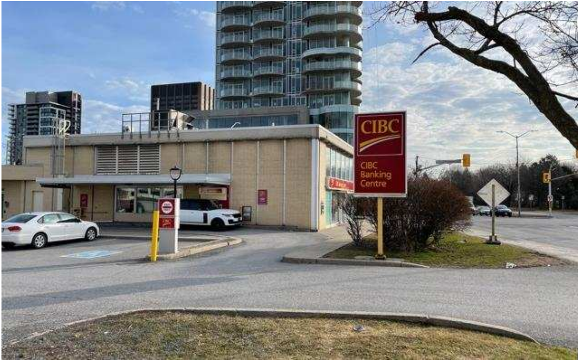
Photograph 3: View of the western side of the subject building. Photograph taken from Carling Avenue, looking east towards Preston Street.
