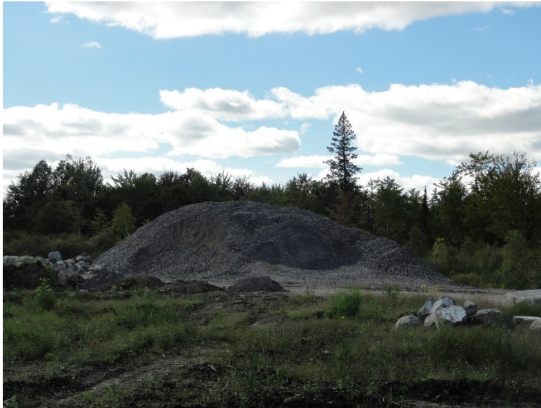
Photo 5 – Stockpile of imported fill consisting of boulders and construction aggregate on the northern portion of the Site, looking northwest.
