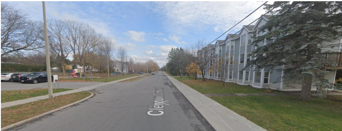
Subject property facing East
