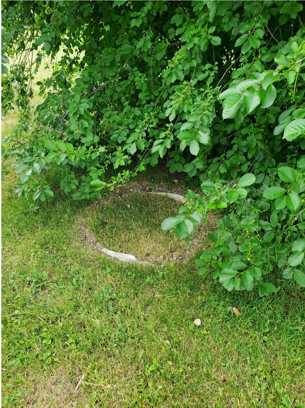
Photo 5: Facing southwest, remnants of a potable well that has been abandoned and backfilled. There are no records of a potable well existing on this site according Ontario Well Records database. The site is serviced by municipal water.
