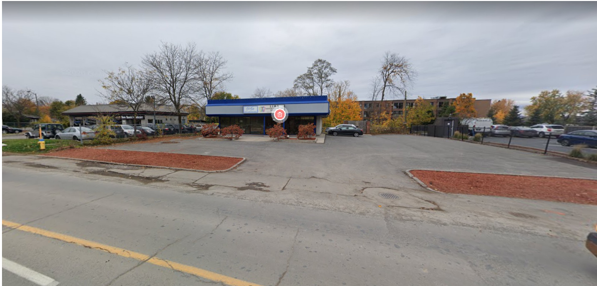
Figure 2. Google Street View of 797 Richmond Rd.
