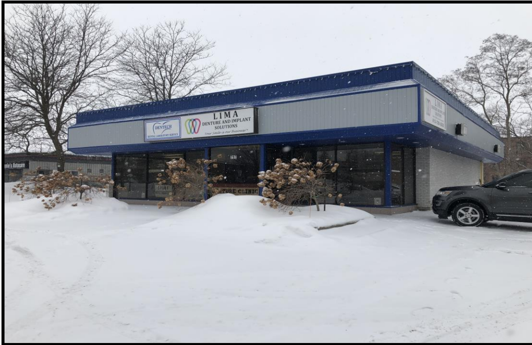
Photograph 1: View of the southeastern portion of the subject site, facing north from Richmond Road.
