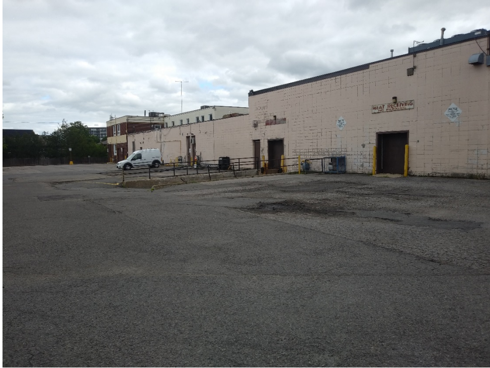
Photograph 3: View of the north side of the Phase One Property looking southeast. View shows the north side of the north commercial building, including the loading dock for the former grocery store and the natural gas meters for the commercial units.
