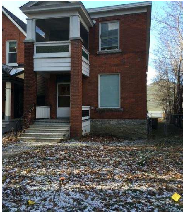
Photograph 3: View of 60 Bayswater Avenue, looking west.
