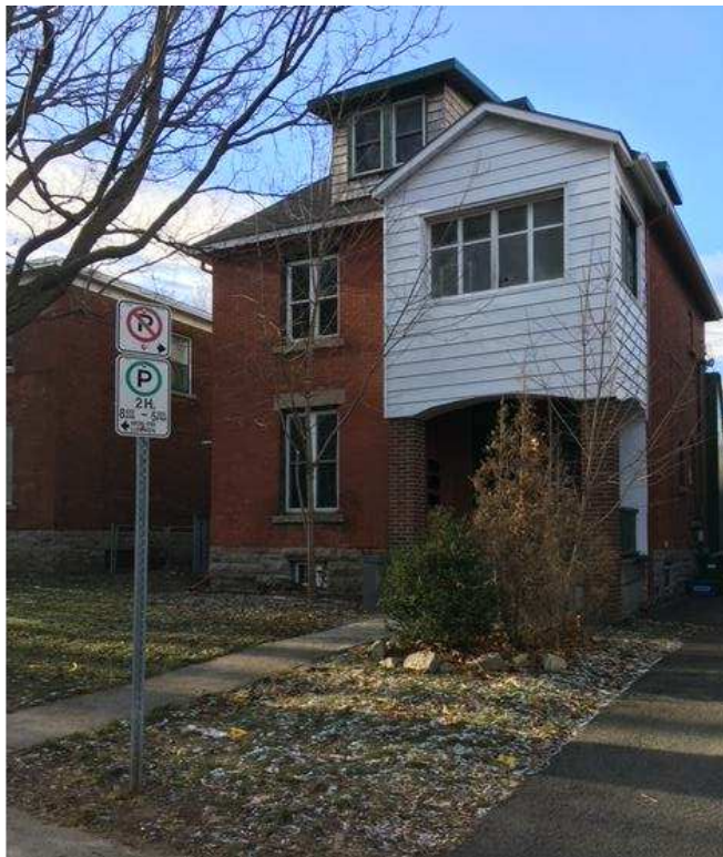
Photograph 2: View of 56 Bayswater Avenue, looking west.
