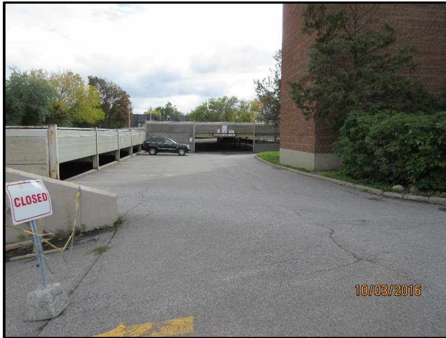
Photograph 3: Photo illustrates the eastern portion of the tower and the parking structure on the northeast corner of the Phase I Property, facing south.
