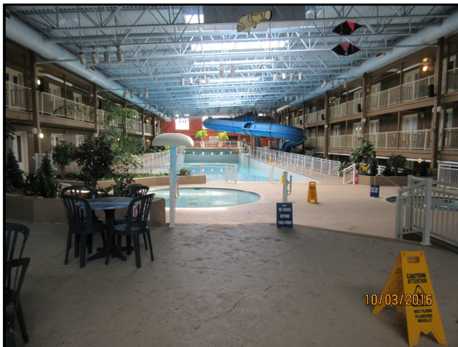
Photograph 12: Photograph illustrates former exterior in-ground pool area which has been retrofitted as an interior water park.
