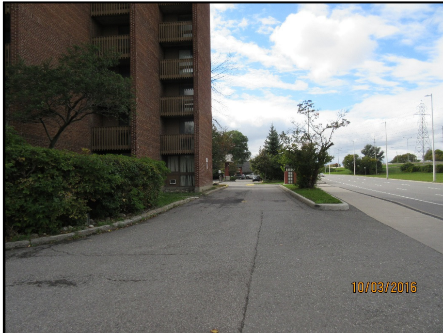
Photograph 2: Photograph shows condemned tower on northeast portion of Phase I Property, facing west.
