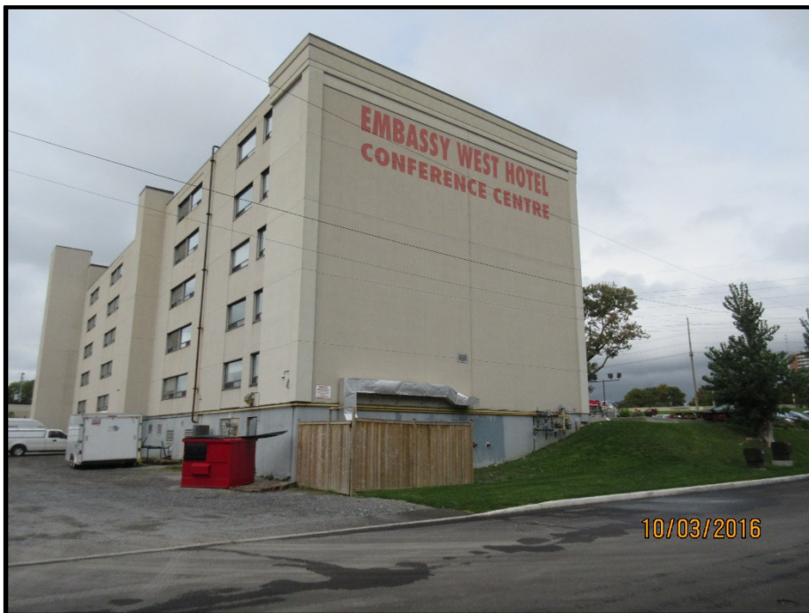
Photograph 14: Photograph illustrates adjacent property to west, across Meath Street, facing northwest.
