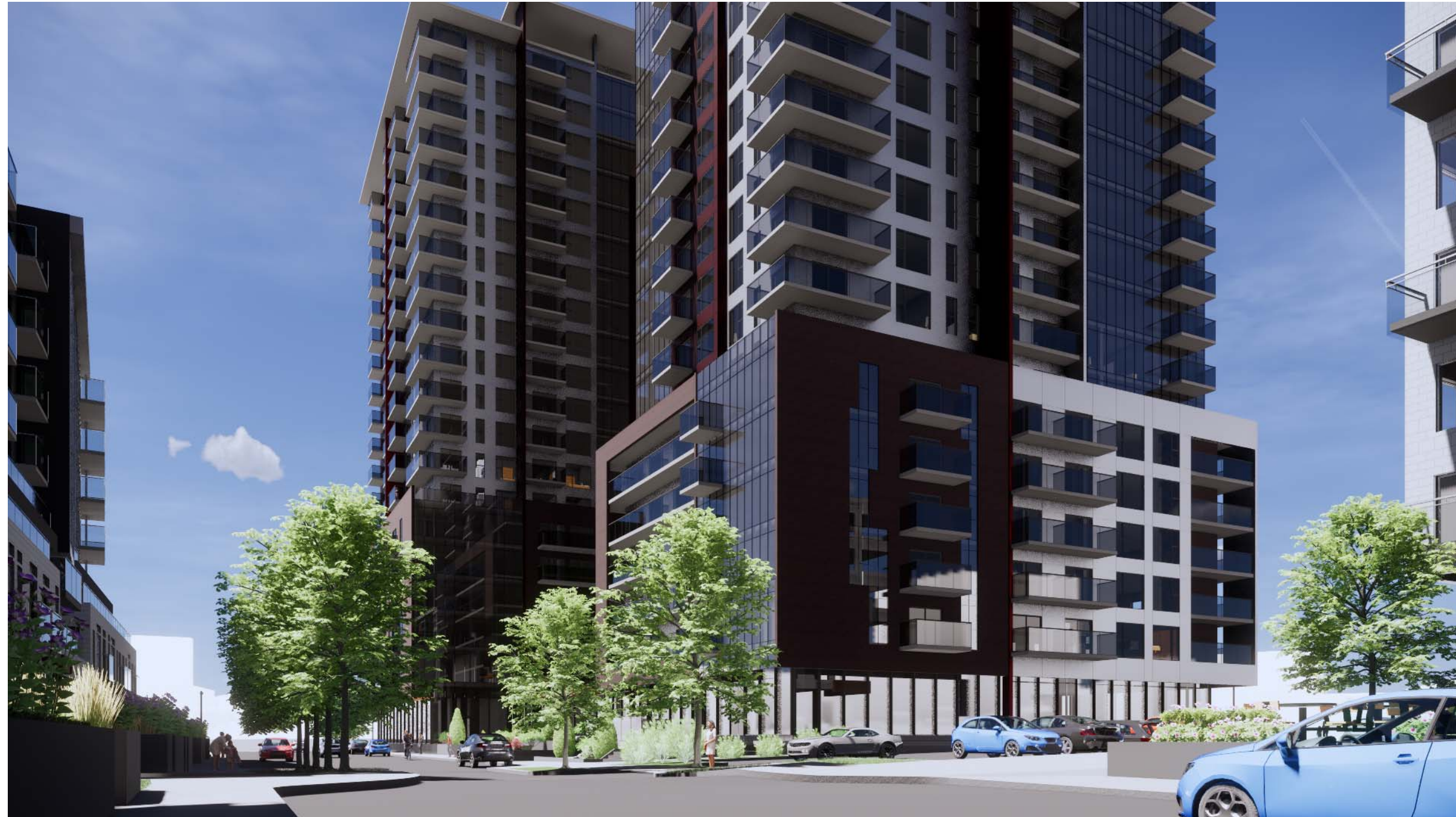
View along interior street : Ground floor commercial with covered walkways.
