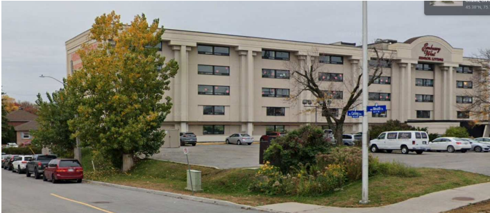
2. VIEW OVER THE EMBASSY WEST HOTEL
