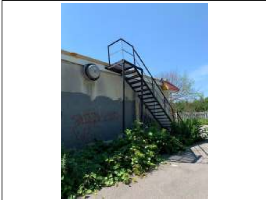
Photograph 3: View of north side of subject building and rear parking lot.
