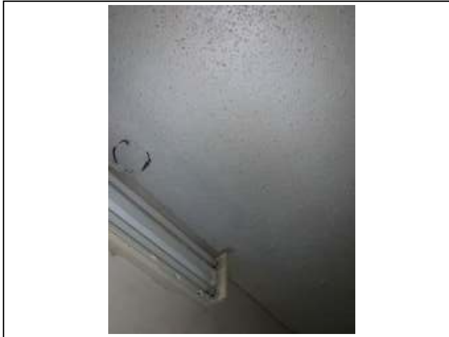
Photograph 27: View of suspected asbestos-containing ceiling stipple throughout the main floor.
