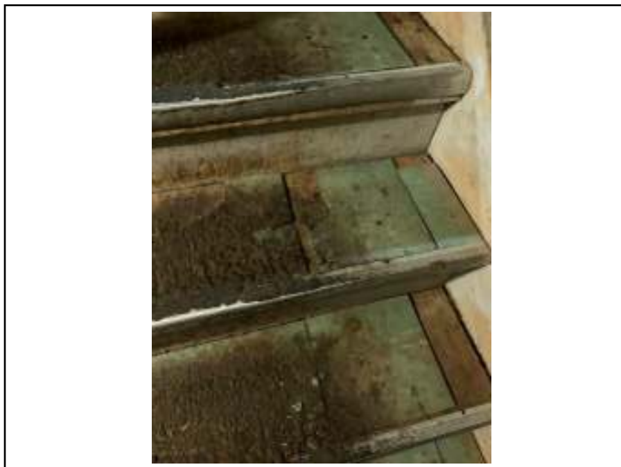
Photograph 22: View of suspected asbestos-containing 9'X9' Vinyl Floor Tile in the basement stairwell.
