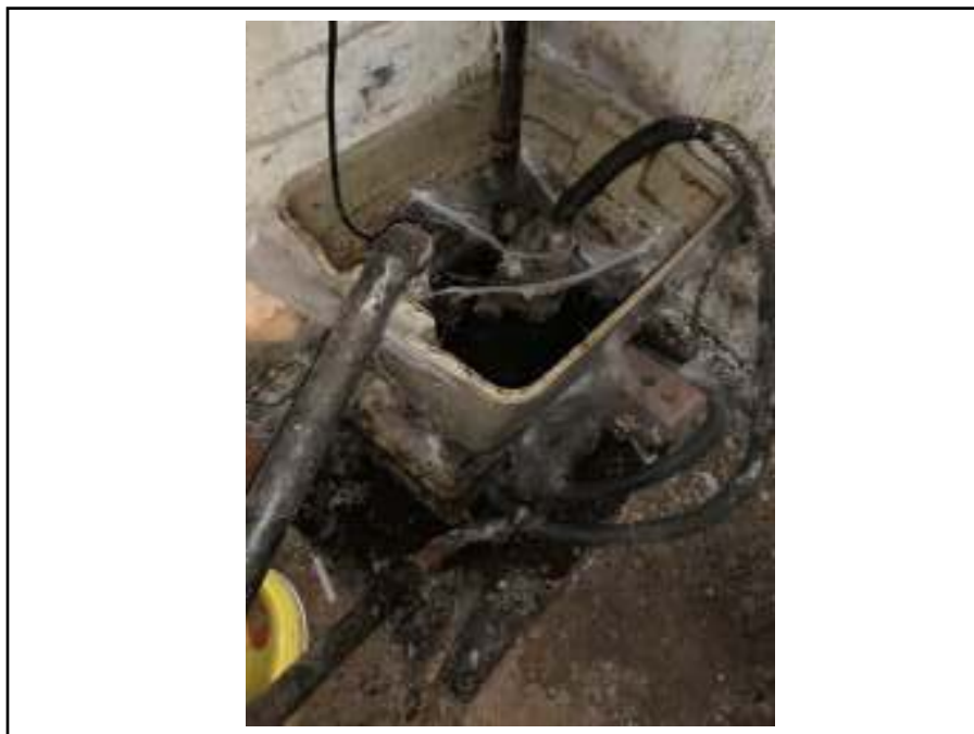
Photograph 18: View sump pit along the south wall of the basement.
