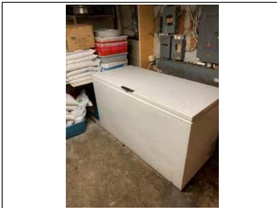
Photograph 20: View of decommissioned chest freezer in the basement, a potential source of ODS
