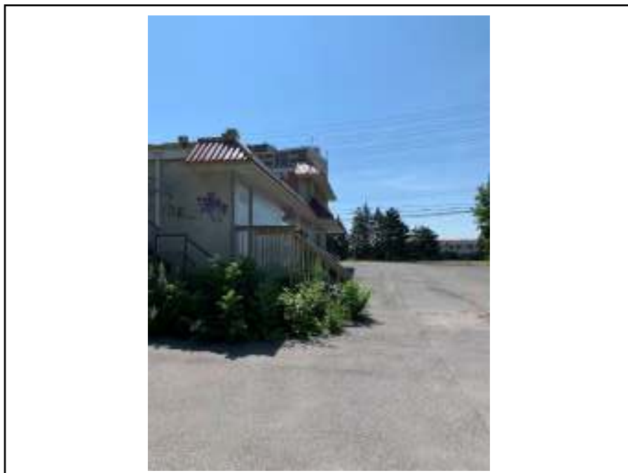
Photograph 6: View of the west parking lot from the north side of the property.
