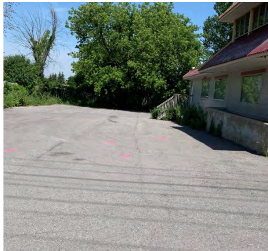
Photograph 2: View of west side of subject building and parking lot.
