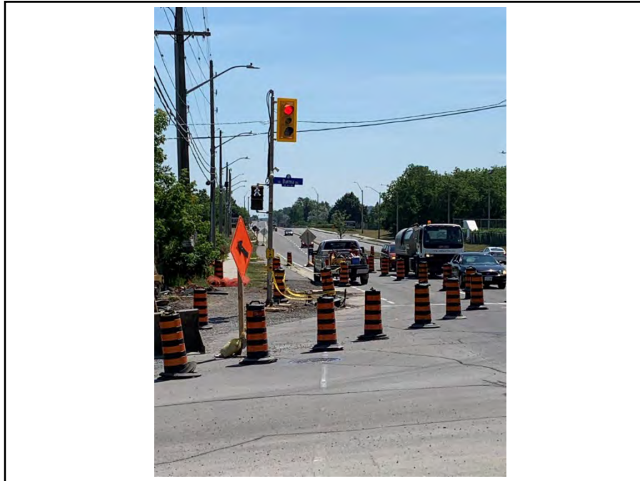
Photograph 45: View of Montreal Road facing east from the intersection of Burma Road and Montreal Road.
