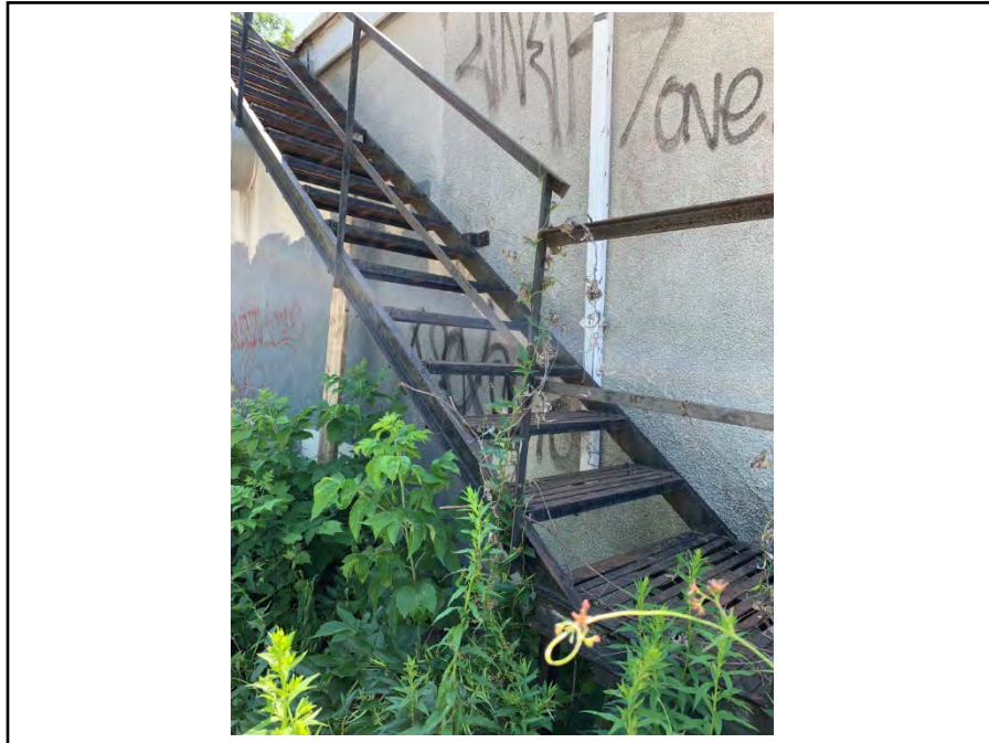
Photograph 7: View of the exterior staircase leading to the second floor unit.
