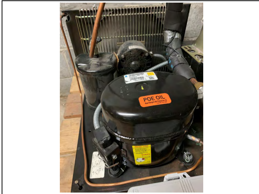
Photograph 11: View of polyester oil tanks in the basement associated with compressors for the walk in fridge/freezer.
