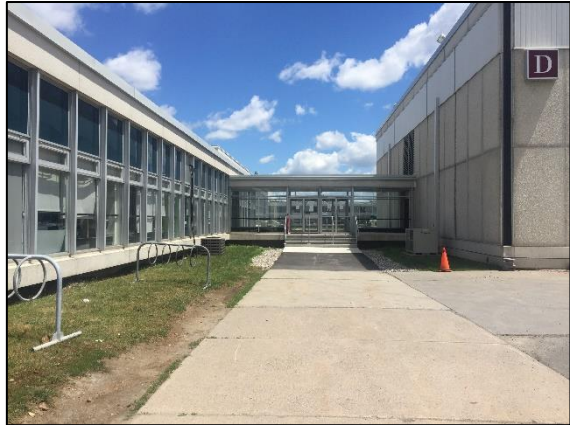
Figure 2-7: View of the Site - Looking East
