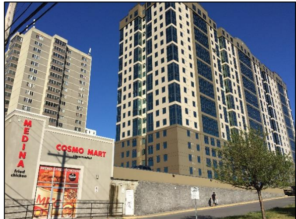
Figure 2-19: View of 170 Lees Ave. Residential Building - Looking South
