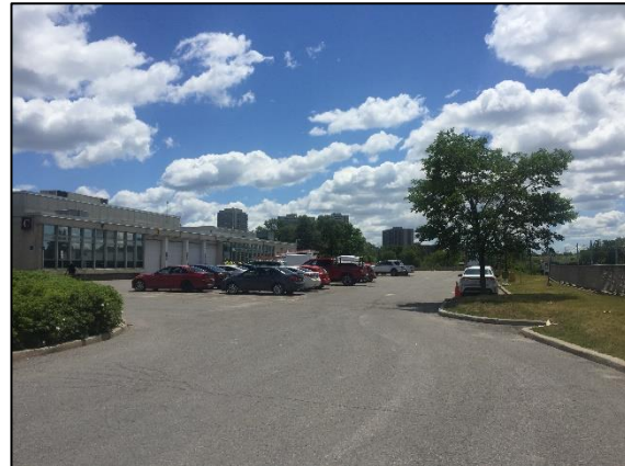
Figure 2-9: View of the Site - Looking Southeast (2)
