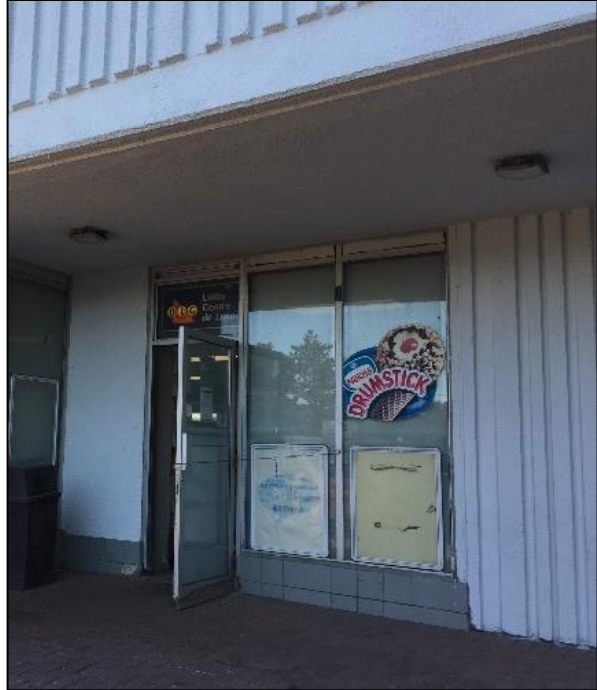
Figure 2-17: View of Lees Market Convenience Store to the West - Looking South
