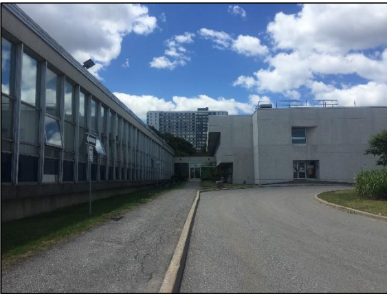
Figure 2-12: View of Building A - Looking East
