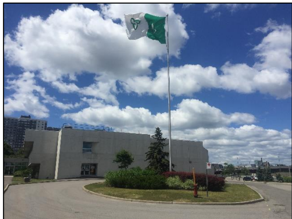
Figure 2-13: View of Building E - Looking East
