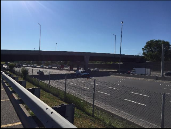
Figure 2-10: View of Highway 417 - Looking North
