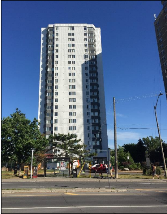
Figure 2-16: View of 190 Lees Ave. - Looking West
