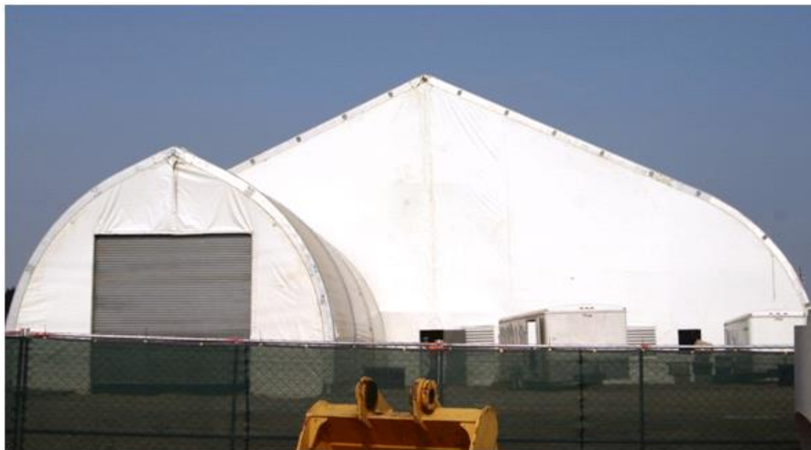
Figure 5.1 Example of a Rigid Structure Used During Environmental Remediation
