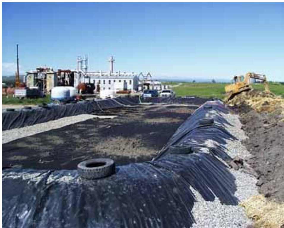
Figure 5.3 Example of Biopile Technology Used to Treat Petroleum Contamination
