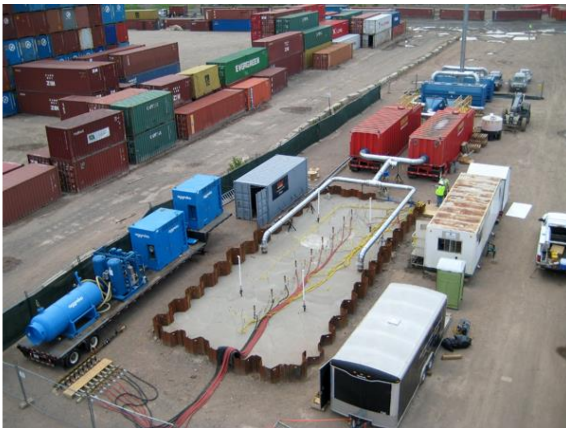
Figure 5.4 Surface Equipment Layout for a Pilot Test of STAR Technology at a Cresol Manufacturing Facility in Newark, New Jersey
