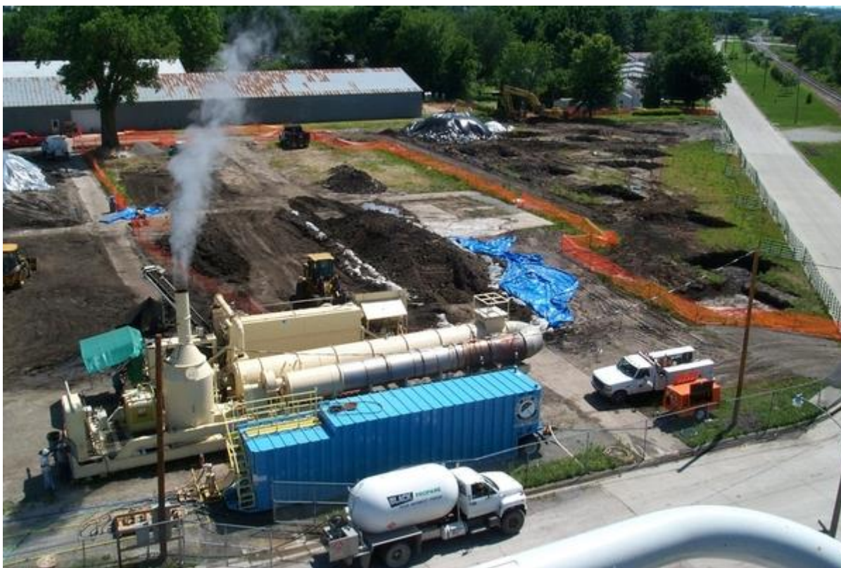
Figure 5.2 Surface Equipment for Ex-Situ Thermal Desorption Treatment
