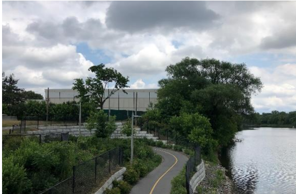
7 - View from Cycle Path Switch Back
