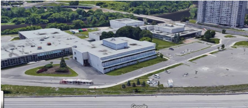
1 - View from North
