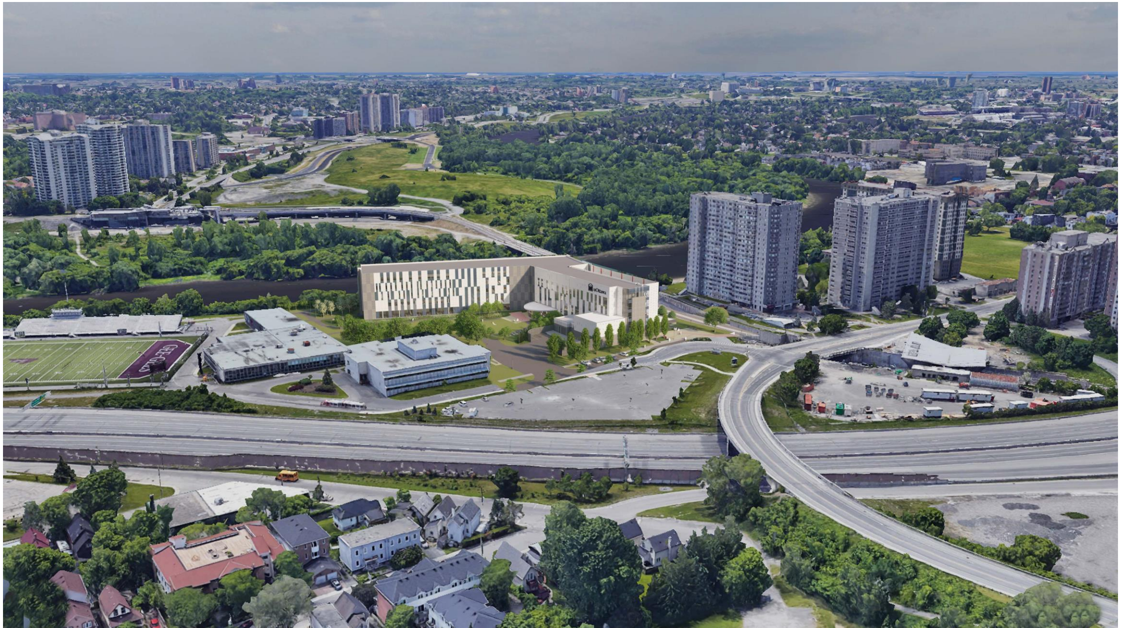
View South / North Elevation
