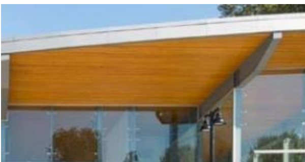
Exposed Wood Soffits on Spine
