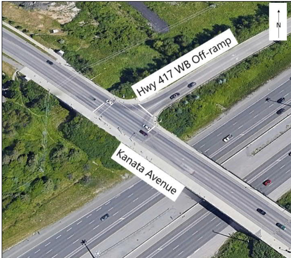
Figure 3.5 Kanata Avenue and Highway 417 Westbound Off-ramp
