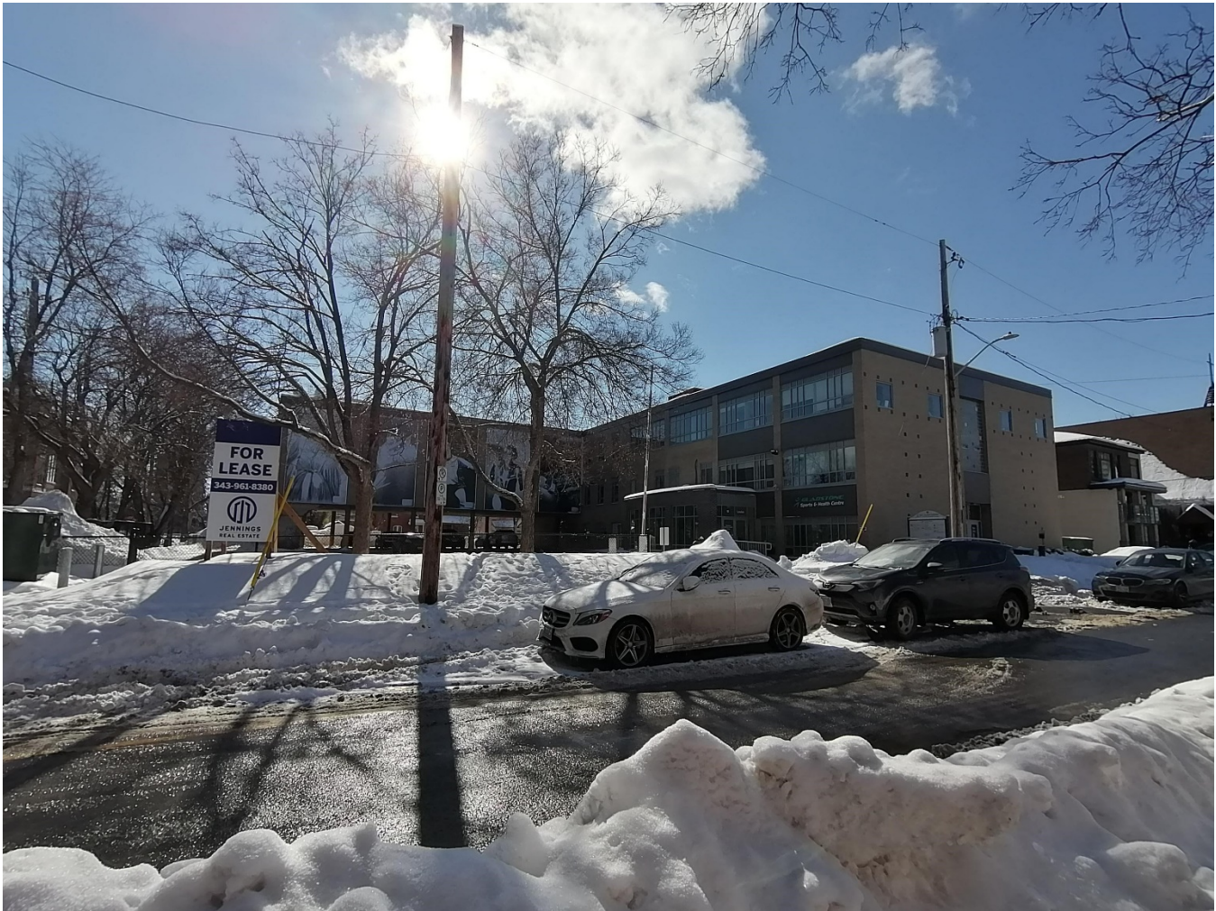
Figure 2: Existing three-storey mixed use building on the subject property
