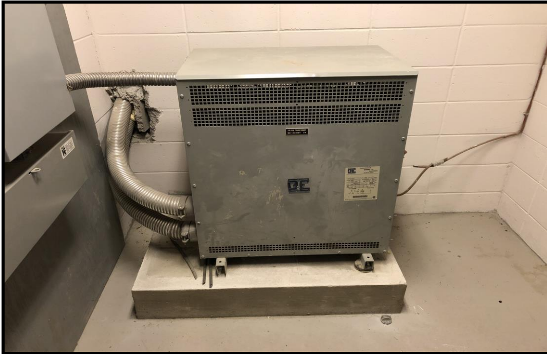
Photograph 5: View of a dry-type, pad-mounted transformer, located within the ground floor electrical room.
