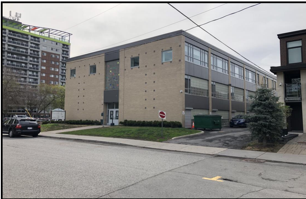
Photograph 2: View of the northwestern portion of the subject site, facing south from Louisa Street.
