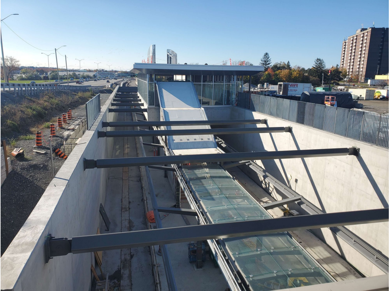
Figure 7: Photo of Pinecrest Station (November 4, 2023) currently under construction
