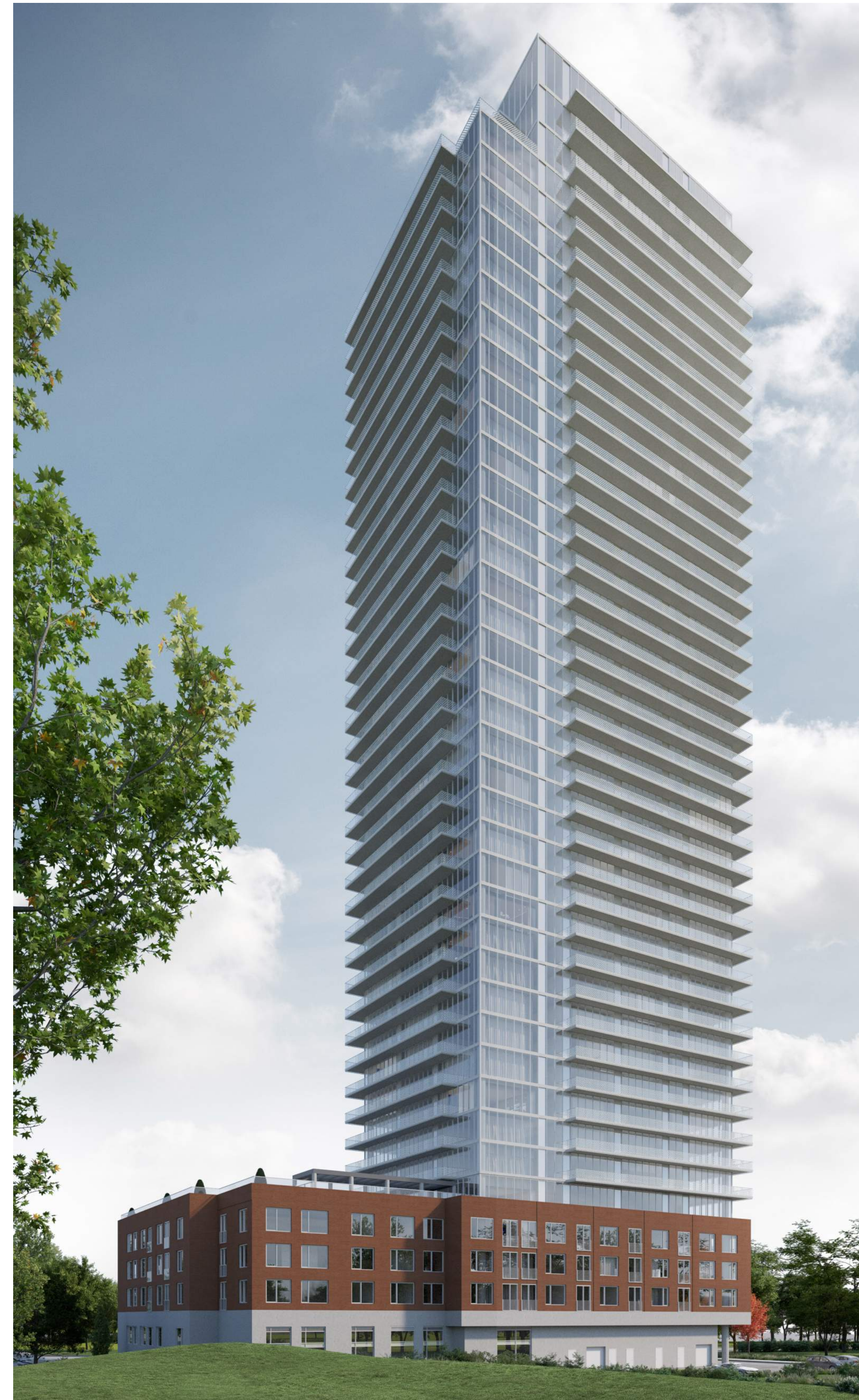
VIEW LOOKING SOUTH-EAST
