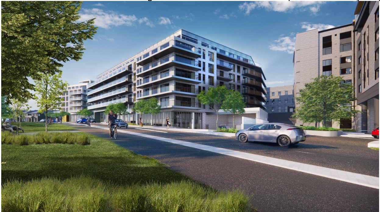
Figure 18. View from Scholastic Drive (east and north façades)
