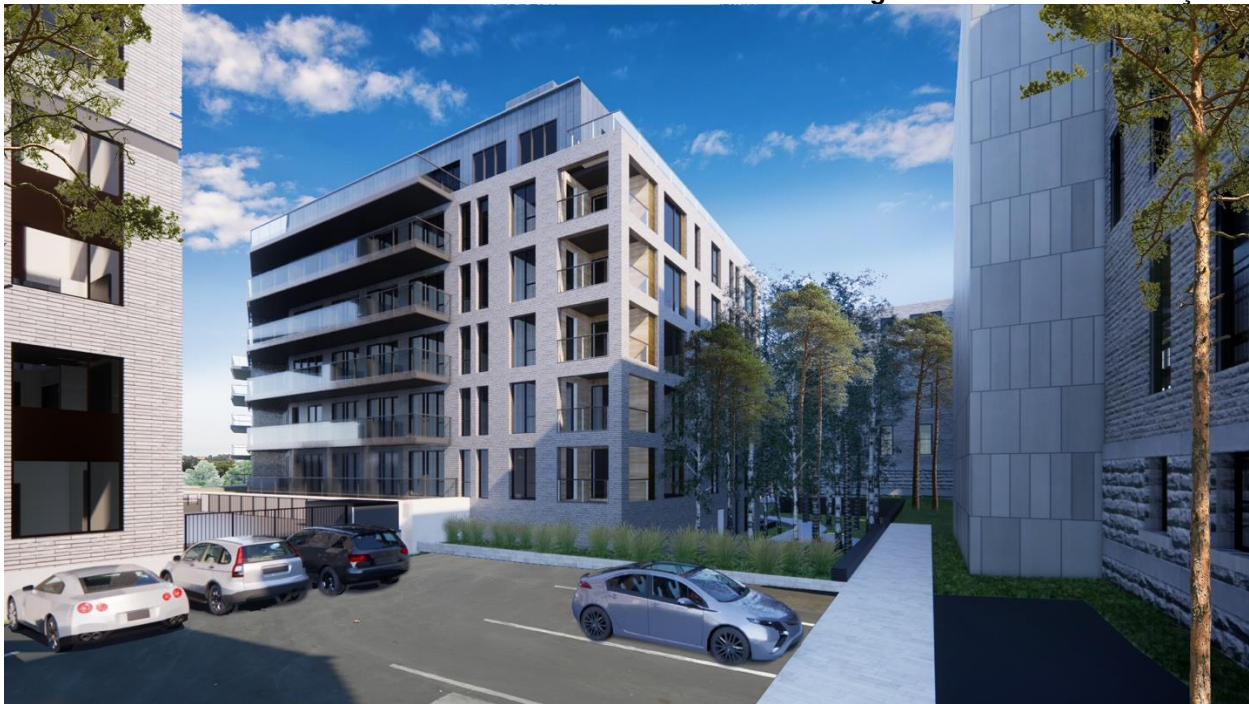
Figure 19. View of north façade
