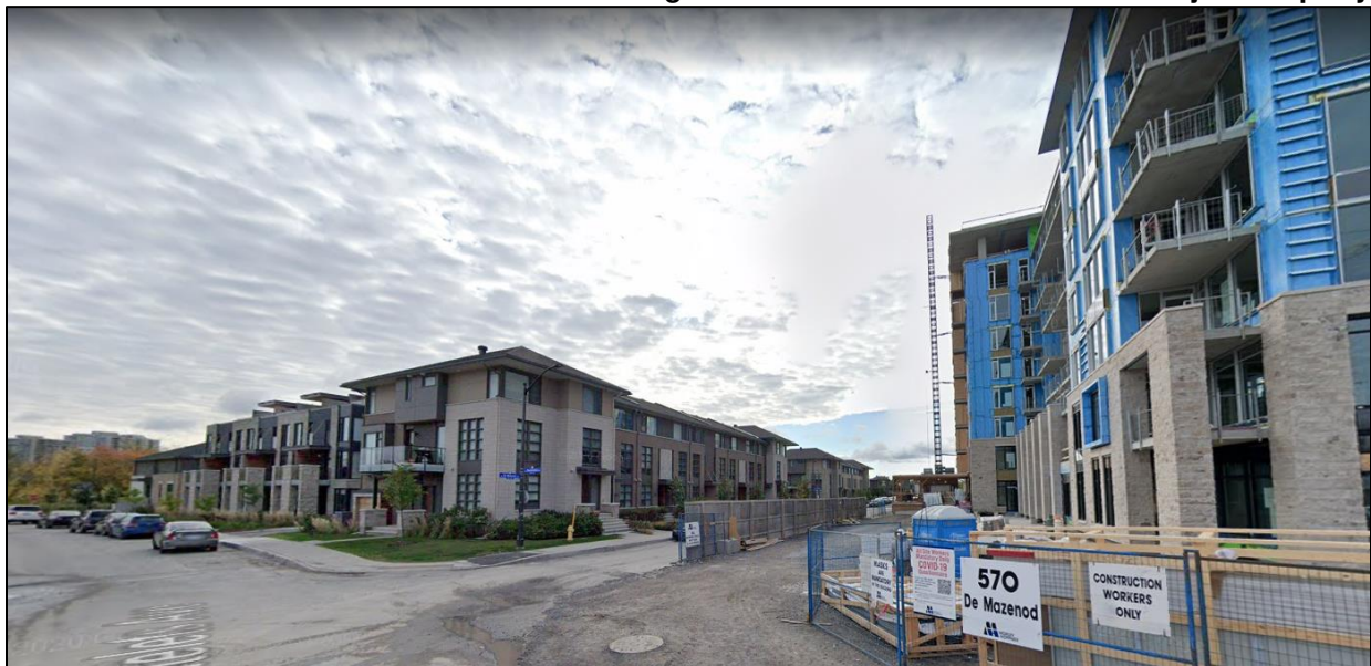
Figure 4. Residential uses south of Subject Property
