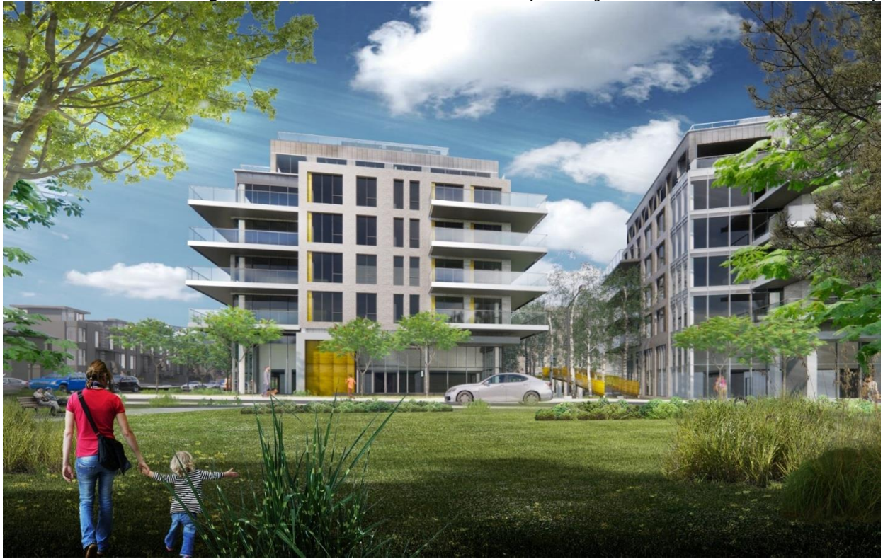
Figure 17. View from Scholastic Drive (east façade and mid-block connection)
