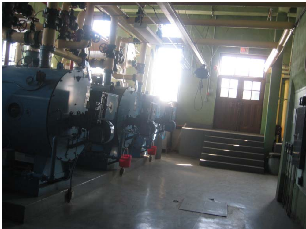
Photograph 14: View of the boiler room.
