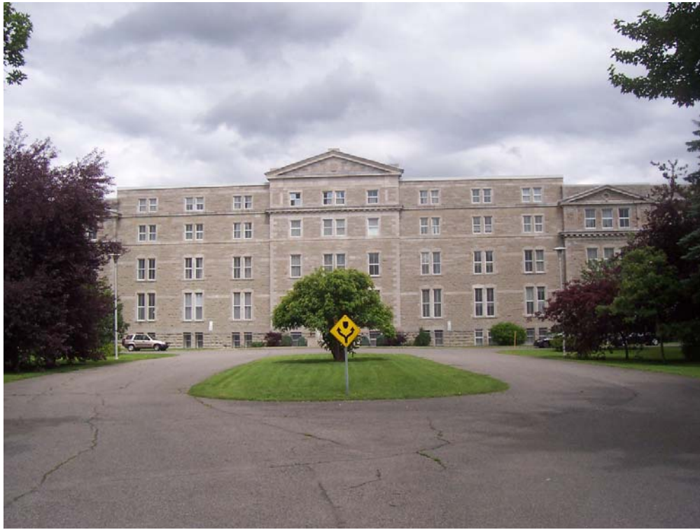
Photograph 1: View of the front entrance of the Site looking east.
