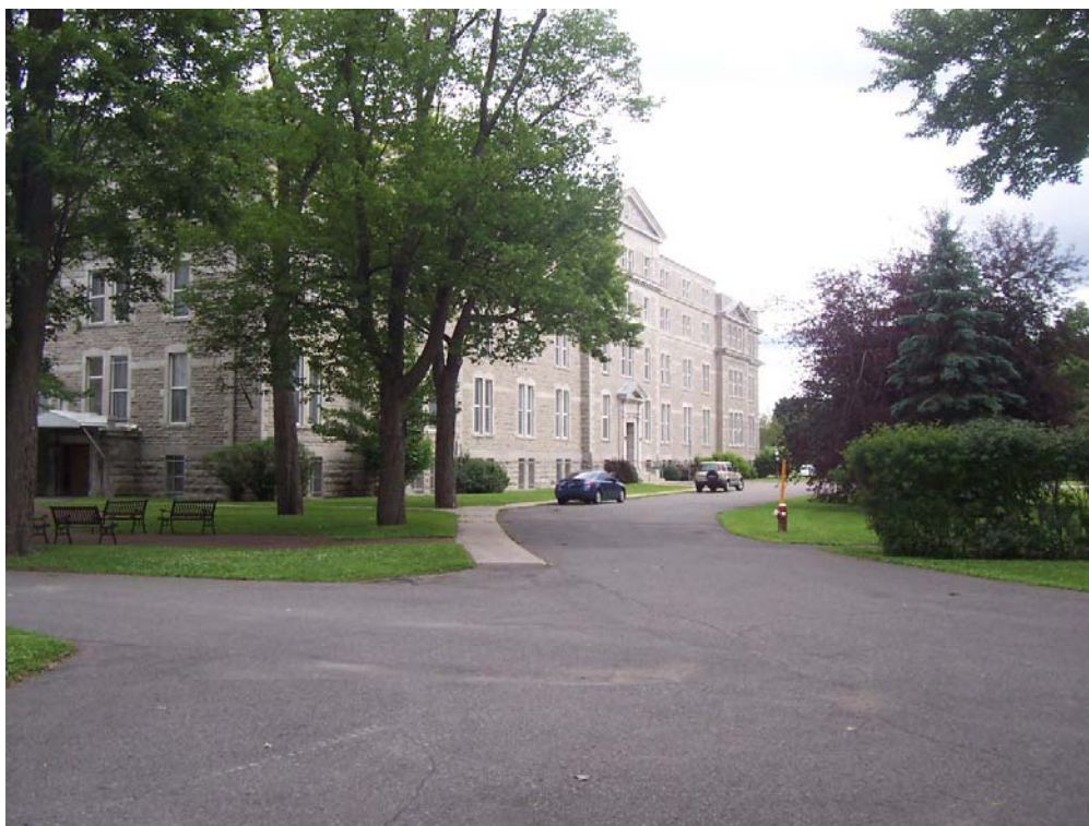
Photograph 10: View of the north part of the Site looking south.
