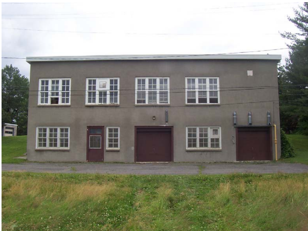
Photograph 12: View of the east facade of the laundry/workshop building looking west.
