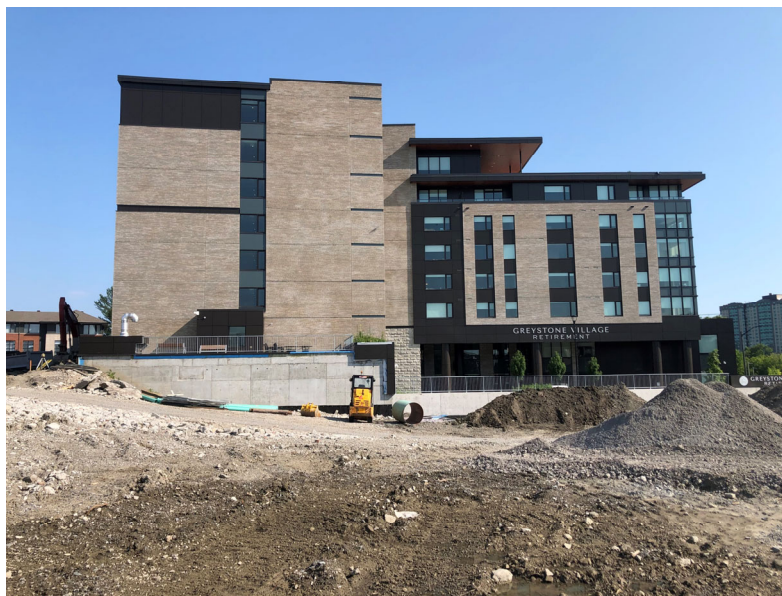
Photo 2 – View of residential building to the north of Site.
