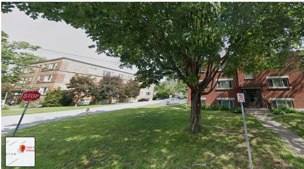
Figure 5: Low-Rise Apartment Dwellings to the North of the Subject Site
