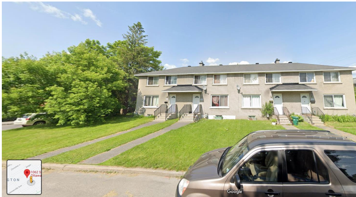
Figure 3: Planned Unit Development to the South of the Subject Site
