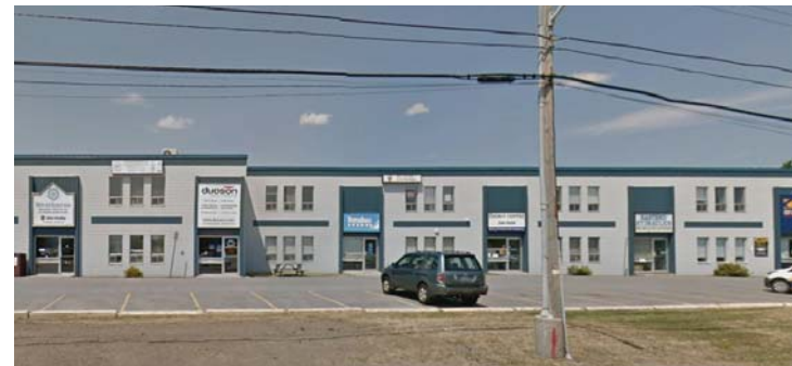
3.2 Two storey neighbouring building on the West
