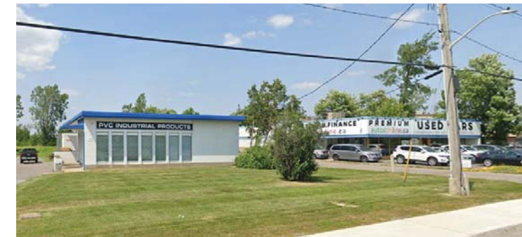
3.3 One storey neighbouring building on the East
