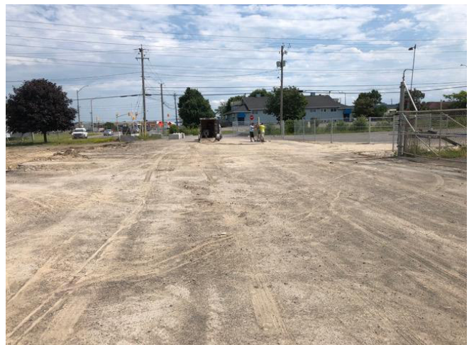
Location of borehole BH6
