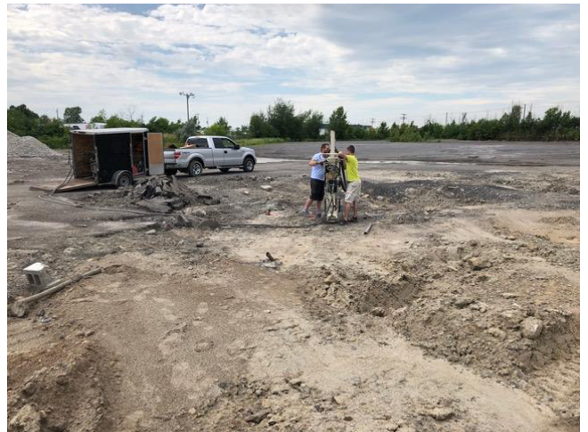
Location of borehole BH4
