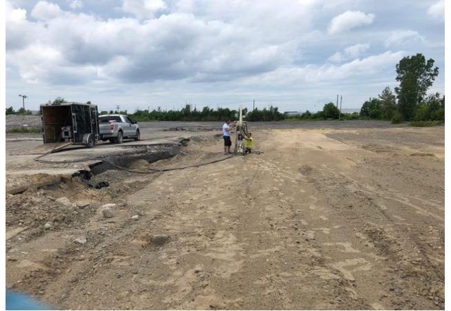
Location of borehole BH8
