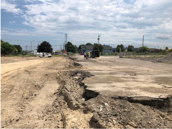
Location of borehole BH13
