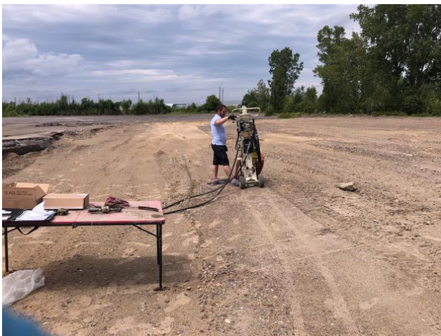
Location of borehole BH5
