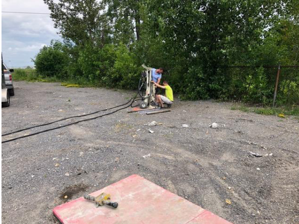
Location of borehole BH1
