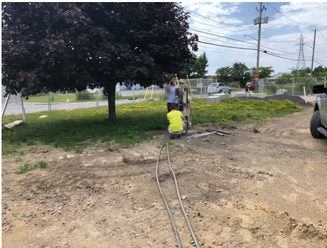
Location of borehole BH11
