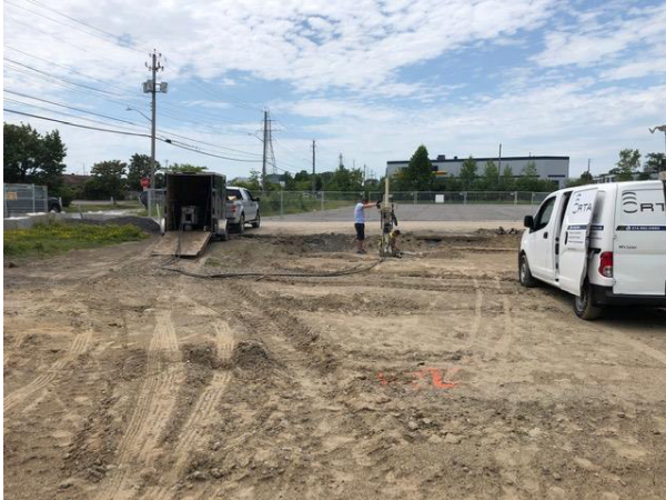
Location of borehole BH7
