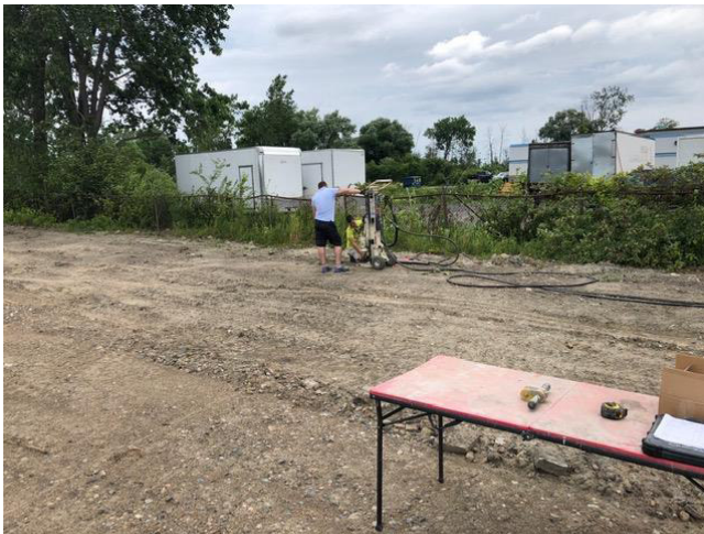
Location of borehole BH3
