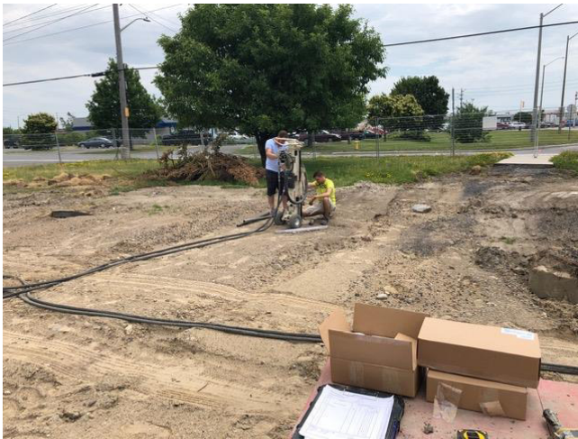
Location of borehole BH9
