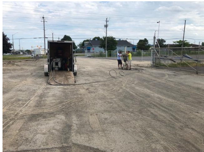
Location of borehole BH12
