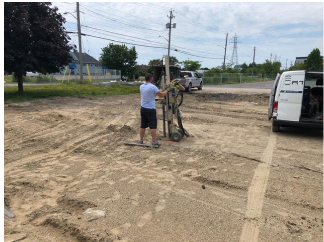
Location of borehole BH10
