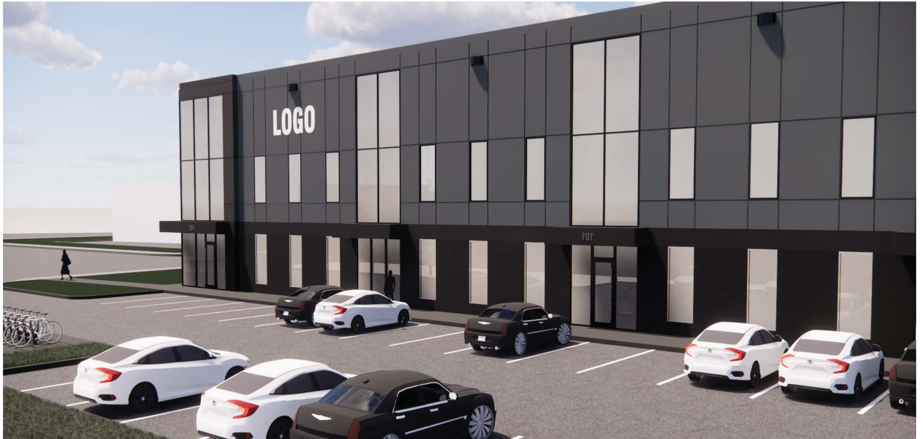
10.1 View of the main entrances. The repetitive pattern of the windows and canopies makes it very easy to subdivide the interior space.
