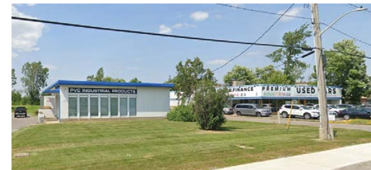
3.3 One storey neighbouring building on the East
