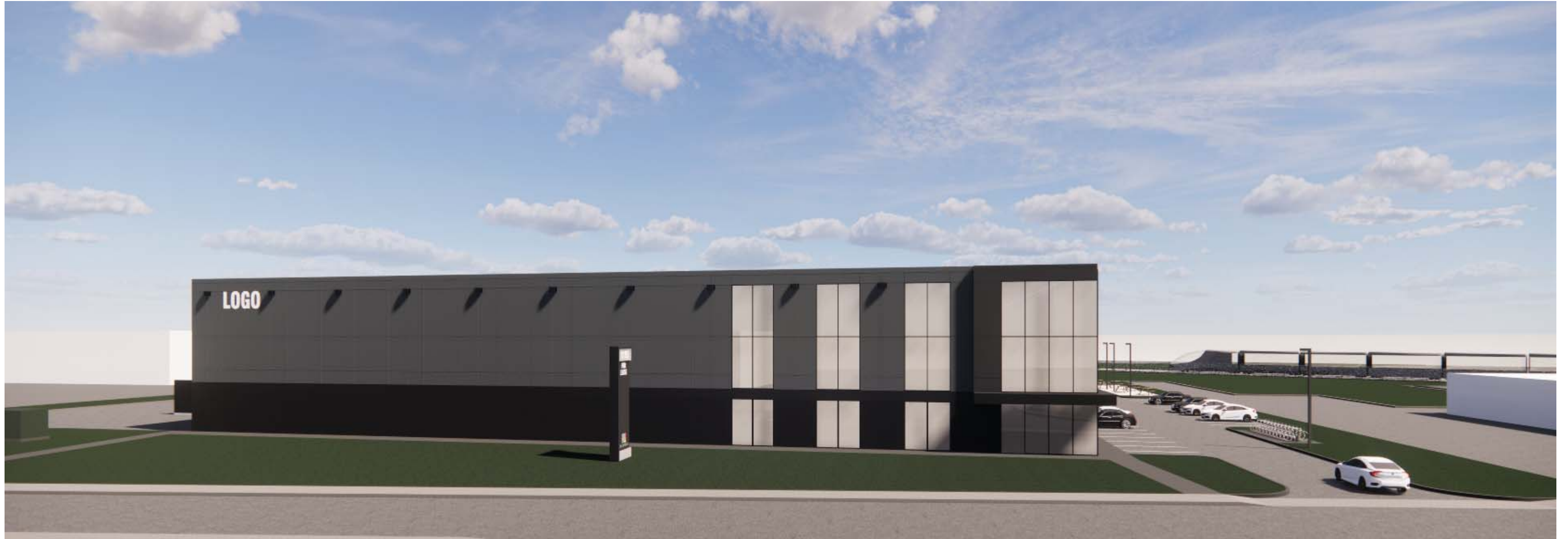
8.1 Facade along Newmarket Street as seen from Bantree Street.
