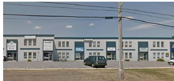
3.2 Two storey neighbouring building on the West
