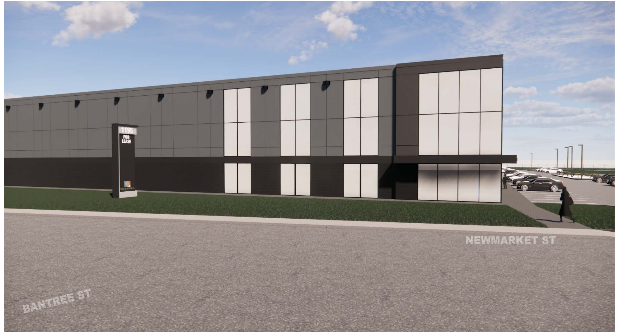
5.1 View of the facade along Newmarket Street, as seen when approaching from Bantree street
